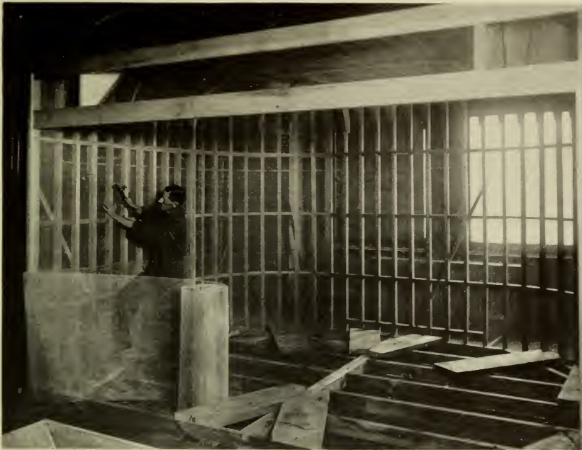
Under structure for a background. Metal may be substituted for wood.
