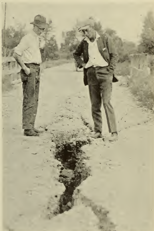
Photograph by Charles C. Mook Above: Trouble for a railroad. This view, taken immediately after the earthquake of July, 1925, at Three Forks, Montana, shows the havoc wrought on a railroad line by the displaced masses of rock loosened by the earthquake
