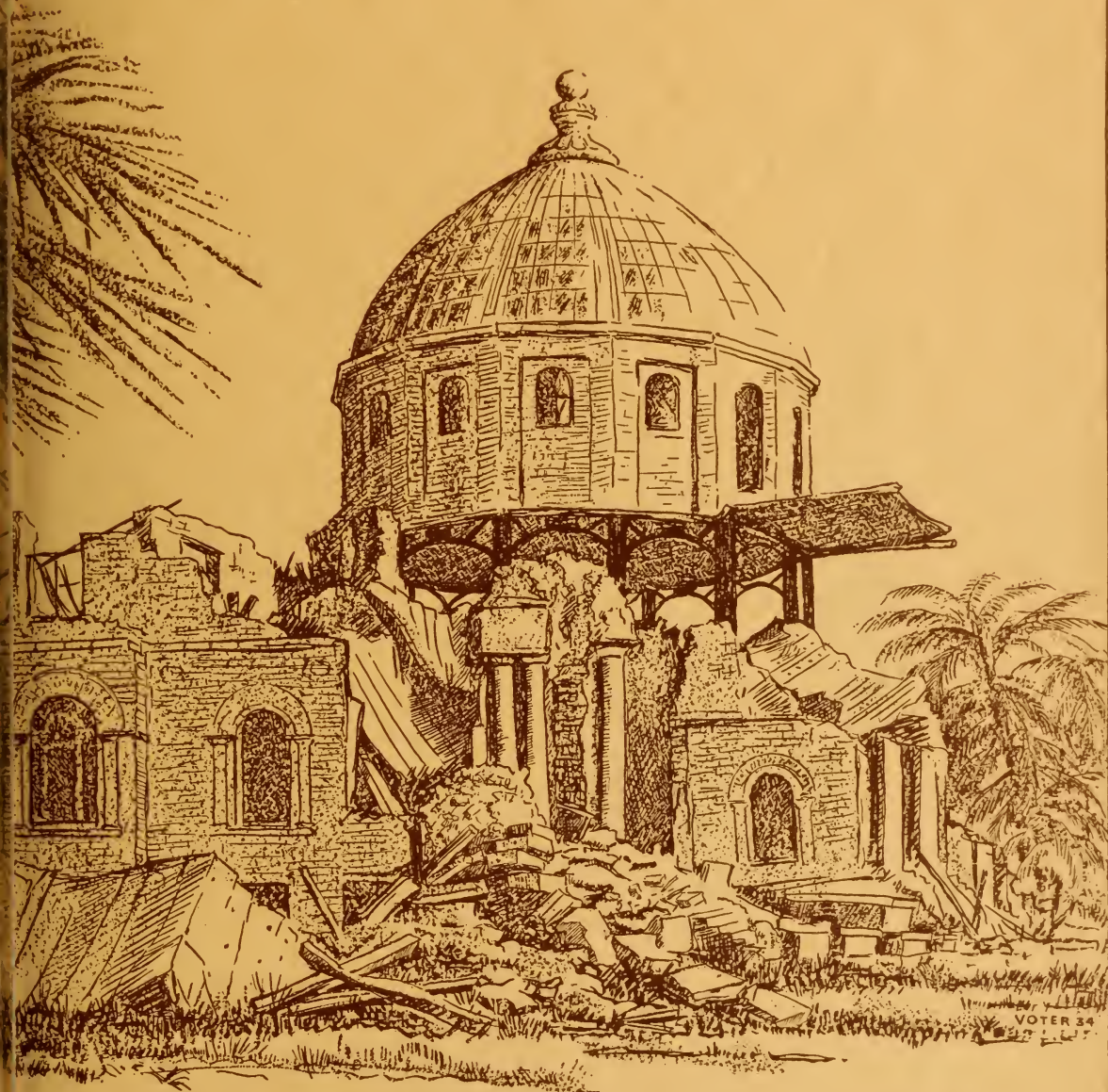
THE LIBRARY BUILDING, STANFORD UNIVERSITY, CALIFORNIA, AS IT APPEARED AFTER THE SAN FRANCISCO EARTHQUAKE OF APRIL 18, 1906
