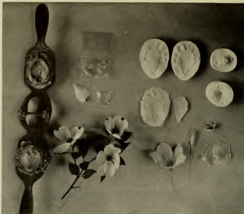
Flowers made of sheet celluloid pressed in metal molds.
