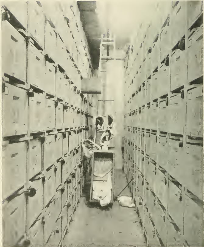
COMMUNITY COLD-STORAGE PLANT, CHICO, SHOWING ARRANGEMENT OF BOXES TO HOLD ONE HUNDRED POUNDS
