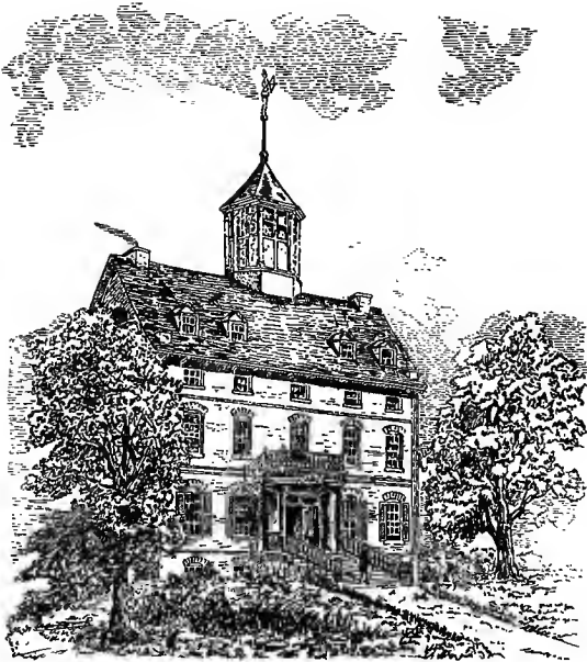
OLD PROVINCE HOUSE.
