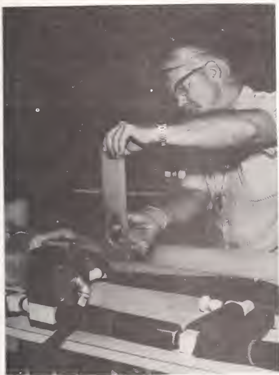
Figure 8. Removing a witness during processing of a large optic.
