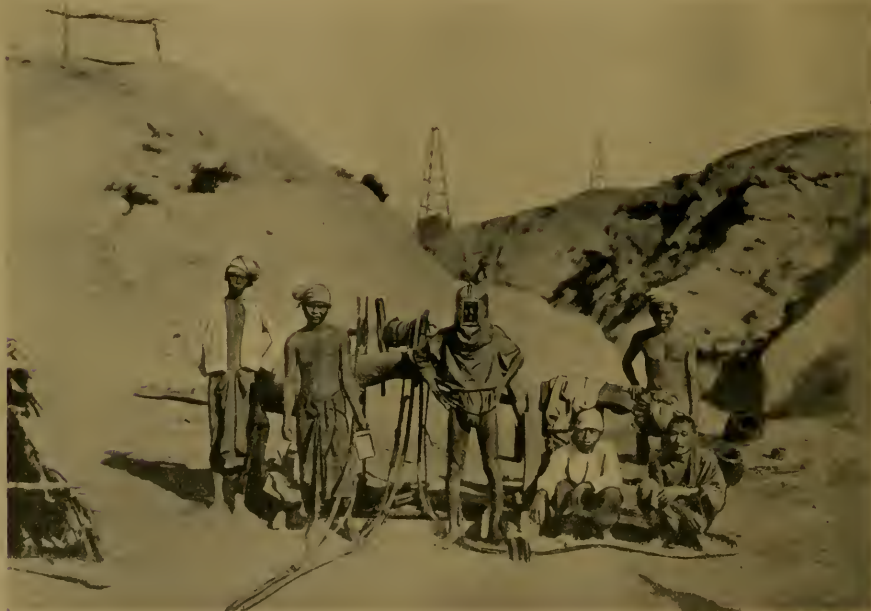
Yenangyaung—Native well-digger in diving dress. (The man on his right is holding the mirror used to illuminate the bottom of the well.) From memoirs of the Geological Survey of India, vol. xli, part i, "The Oil-fields of Burma."
