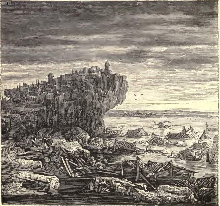
AFTER THE EARTHQUAKE.
