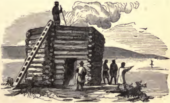
LIGHT-HOUSE AT GHIJIGA.
