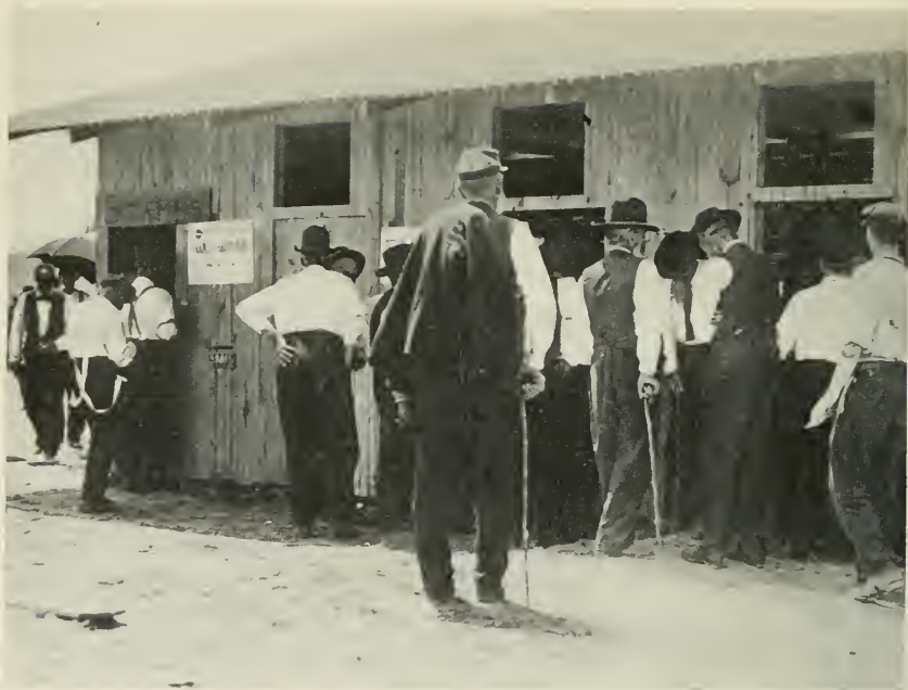
U. S. TEMPORARY POST OFFICE IN THE GREAT CAMP.
