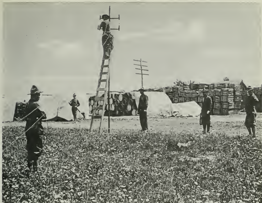
SIGNAL CORPS BUSY.
