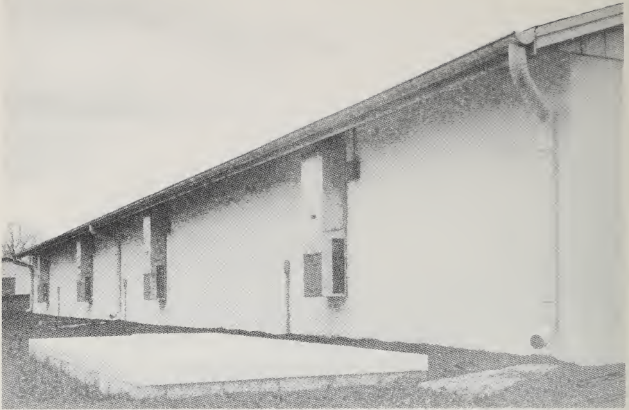
Side view of farrowing house at the University of Kentucky, showing four of the eight electric heat pumps that were donated by East Kentucky Power cooperative.
