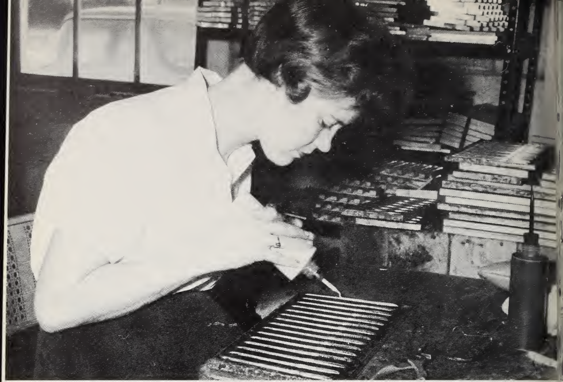
Employee at bait factory squeezes plastisol into mold—first step in making flexible plastic bait. These night crawlers will be fitted with hooks, then baked.
