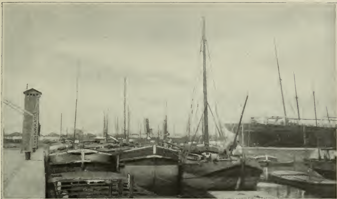
The clustered barges that float away to France and Holland.
