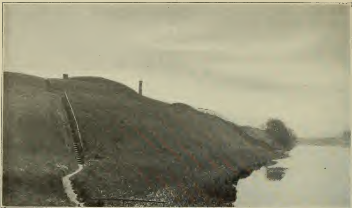
A bit of the fortifications which are being removed to make room for more docks.
