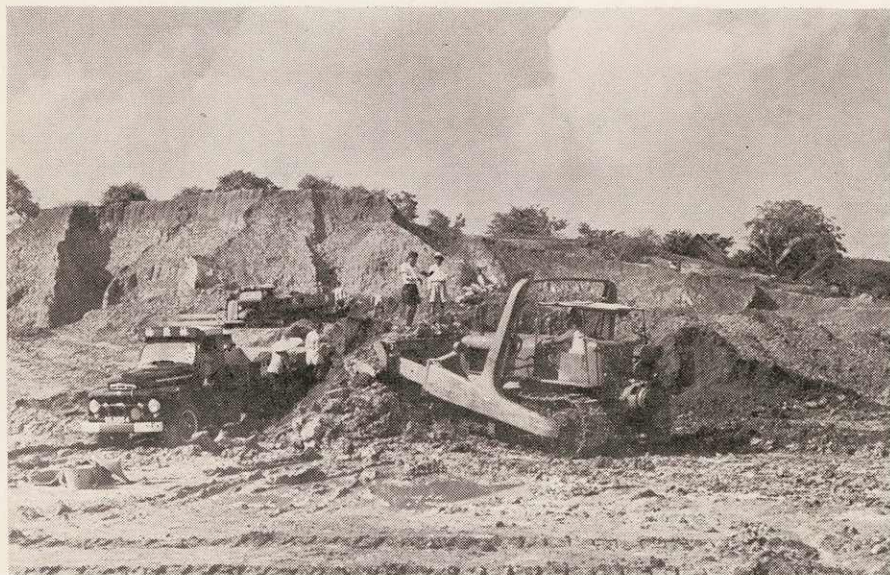
Preparation of building site at Tiong Bahru (South)
