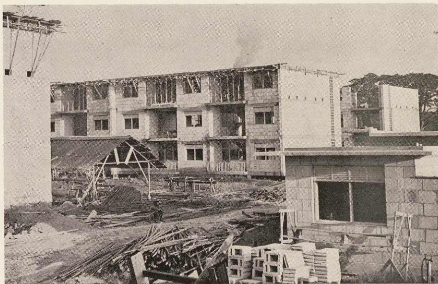
Part of eighteen blocks of flats under construction at Alexandra Road
