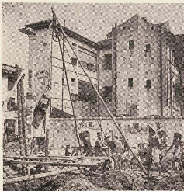
Bakau Piling for S. I. T. Tenements at Albert Street — Old Method.
