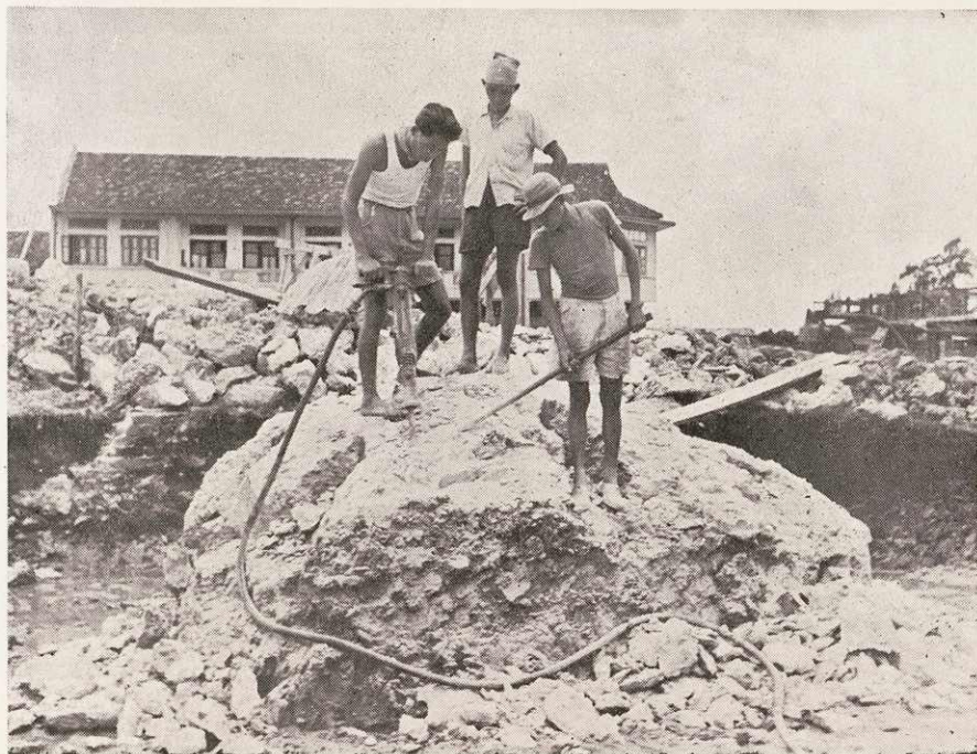
Demolishing old foundations at Jalan Besar (North)
