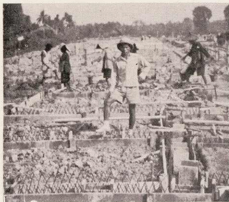
Placing Foundation Beams.
