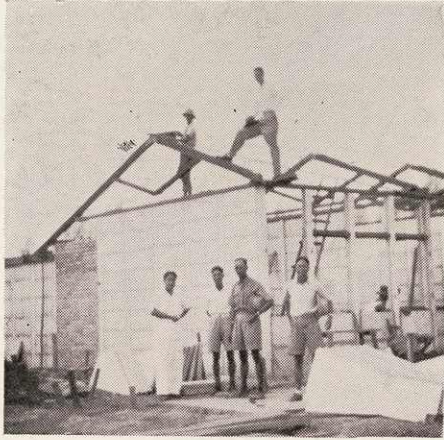
Erecting Trusses.
