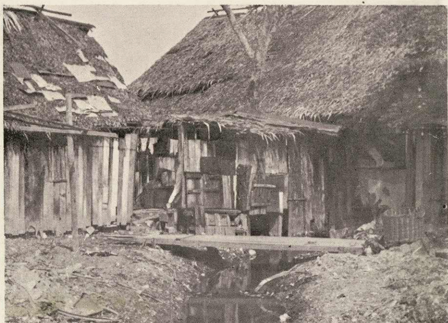
Covent Garden. Latrine over Drain.
