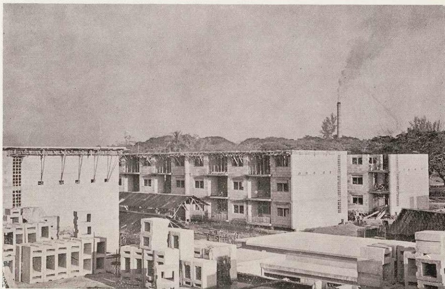
Flats in course of erection at Alexandra Road
