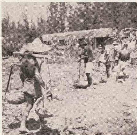
Clearing and Excavating Site.
