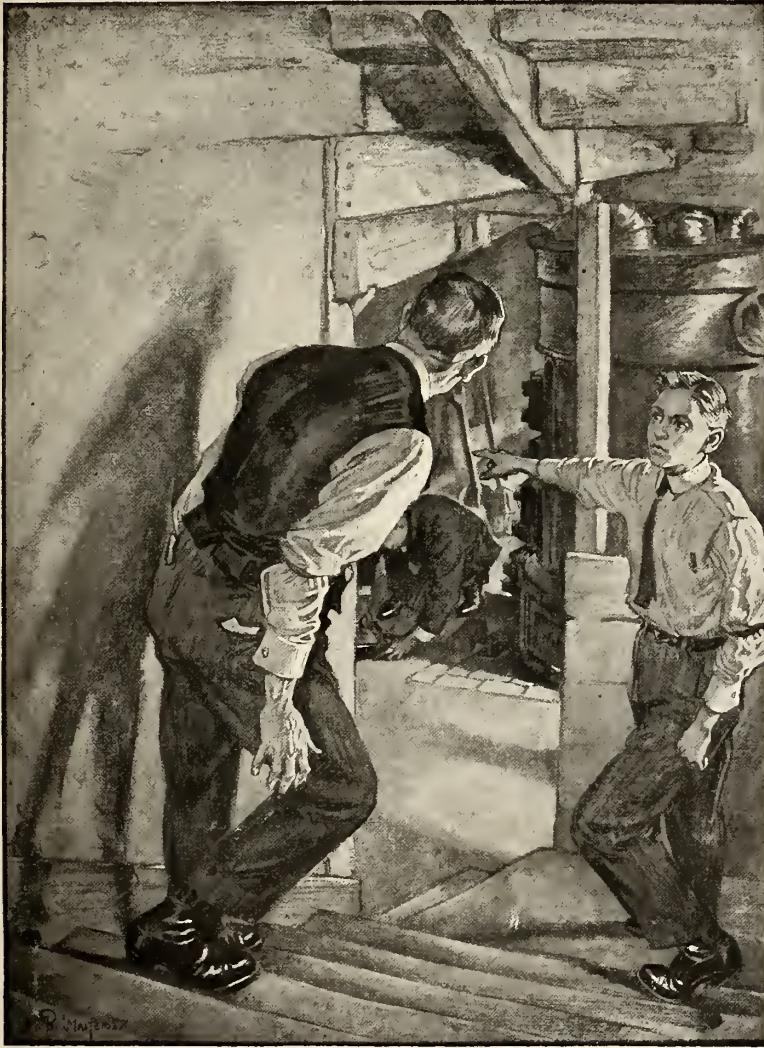
"QUIETLY THEY TIPTOED DOWN THE CELLAR STAIRS."
