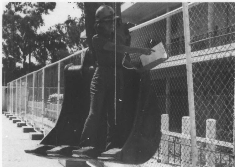
Deborah Jones at construction site on the embassy grounds.
