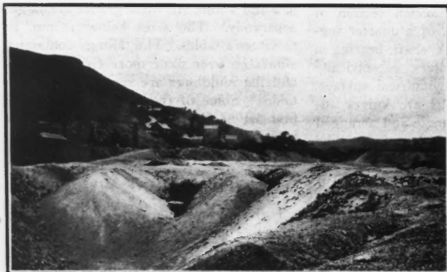
PUMPING AND HAULING SHAFTS, MINERA MINE
