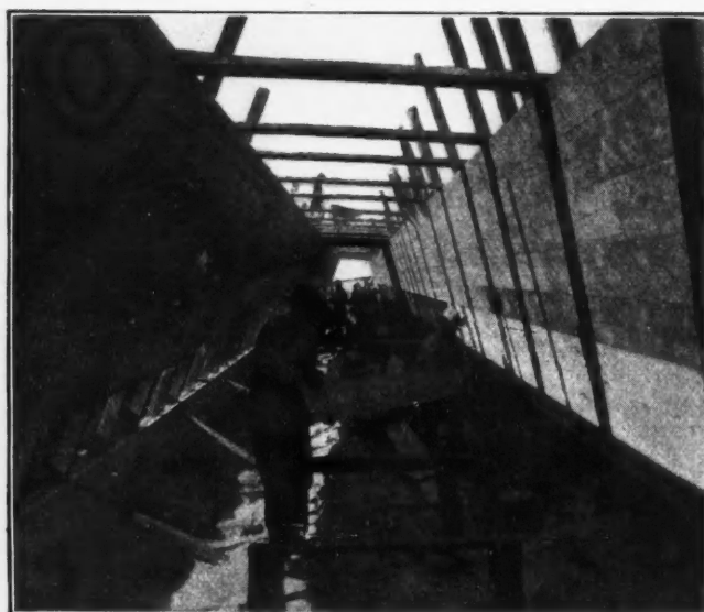
INSIDE THE FORM FOR CONCRETE-MORTAR BLOCK
