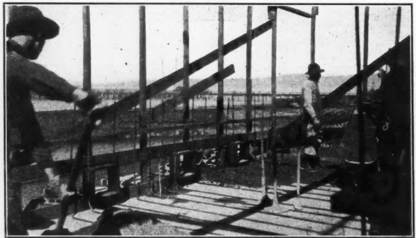
LAYING FLOOR OF INLET FLUE
