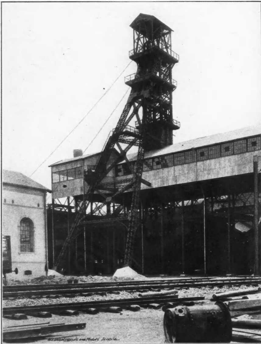
HEADGEAR AT SHAFT NO. 3, AUBONÉ
