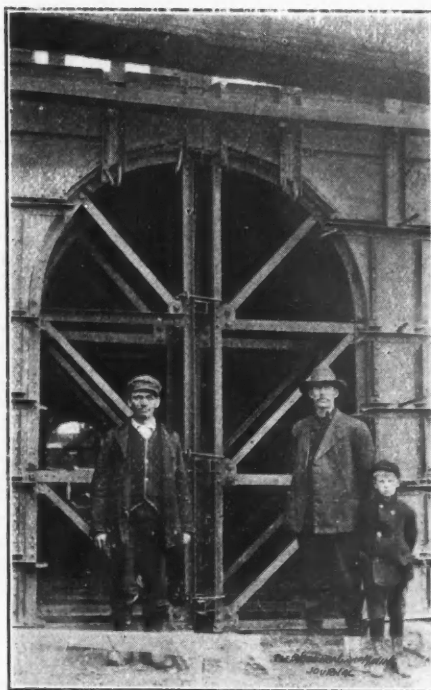
FORMS FOR SLAG CULVERT AT BUTTE REDUCTION WORKS
