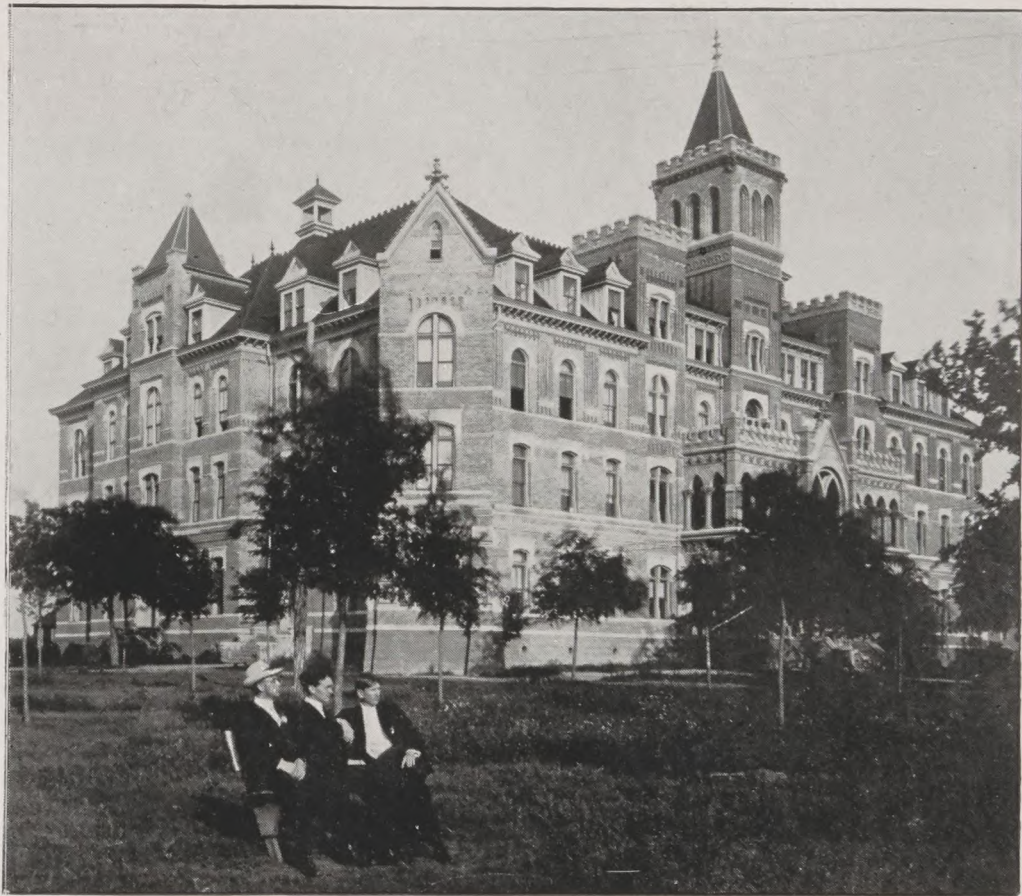
NORTHEAST VIEW OF BUILDING.
