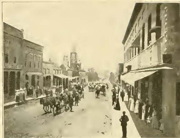
FIG. 63. In the business district of Batesville. A view in Main Street.
