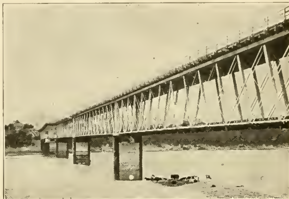
FIG. 9. One of the great bridges spanning the Arkansas River at Little Rock.
