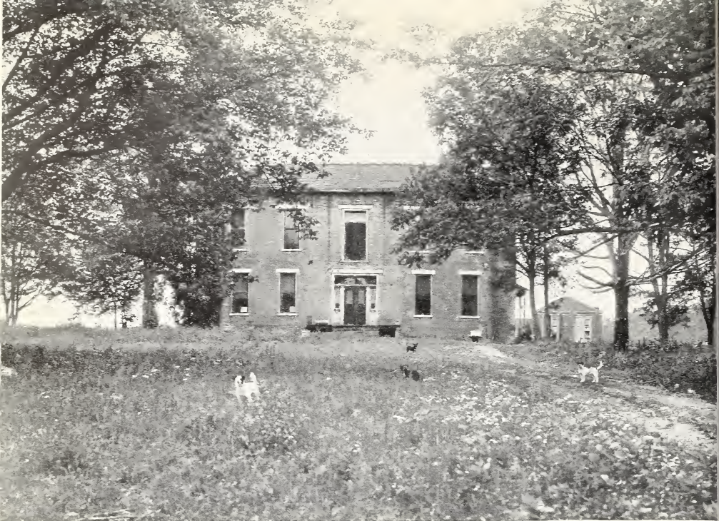
FIGURE 7.—Even a well-designed and well-built farmhouse EXT- deteriorates under absentee ownership.
