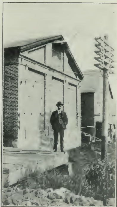
Rosland, Central Transformer Station 60,000 V. — 20,000 V.
