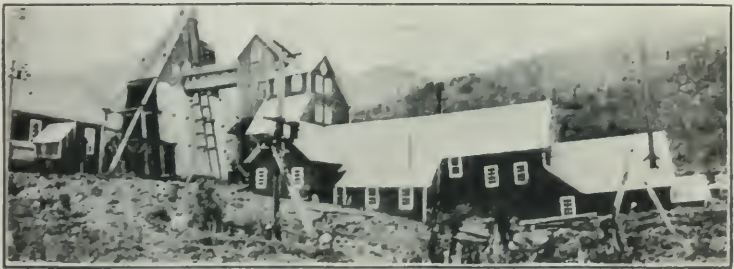
Compressor and Hoist House
