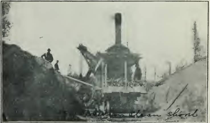
Marion Steam Shovel.
