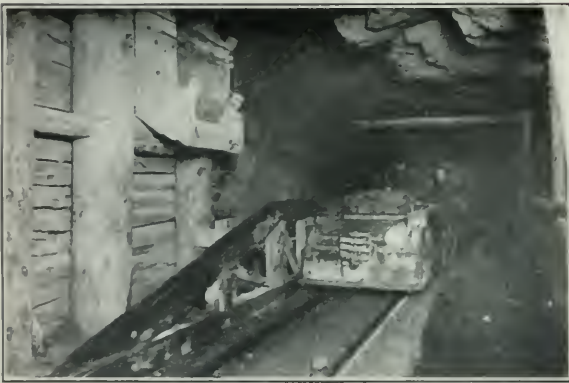
Fig. XIV—Ore Train approaching Pocket. The incline for dumping the cars is shown on the left.
