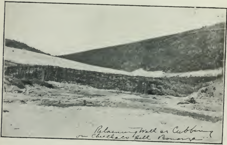
Retaining Wall and Cribbing on Cheechaco Hill, Bonanza.
