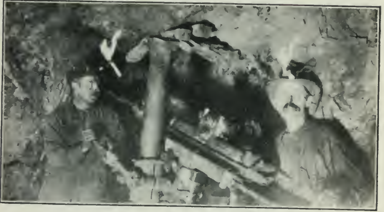
Machine Work (Underground).
