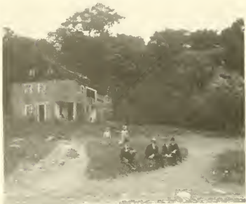
STONE HOUSE, BRADY TOWNSHIP
