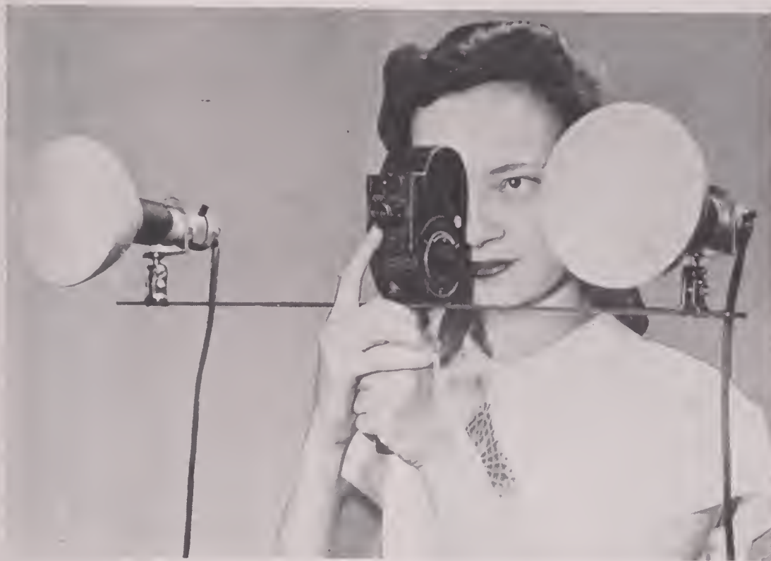
Pictured above is the handi-bar movie light, recently added by the Bell & Howell Company, Chicago, to its line of movie accessories. Whether the handi-bar is used with or without a tripod, individually-controlled light sockets mounted in swivels at either end may be swung with the camera or pointed in any direction that suits the operator. Either photoflood reflector bulbs or spotlight bulbs may be used to furnish illumination.
