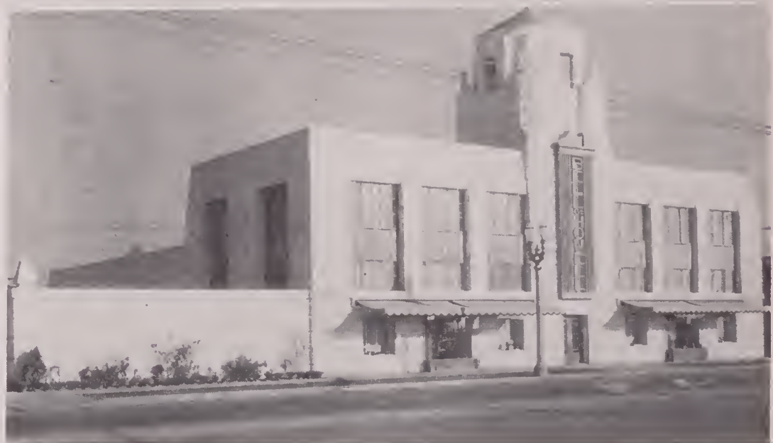
(At top) Early plant of Bell & Howell on Larchmont Avenue, Chicago. (Center) The new Lincolnwood Laboratories, latest of the three plants in the Chicago area. (Bottom) Company's Hollywood Laboratories which service the motion picture studios.
