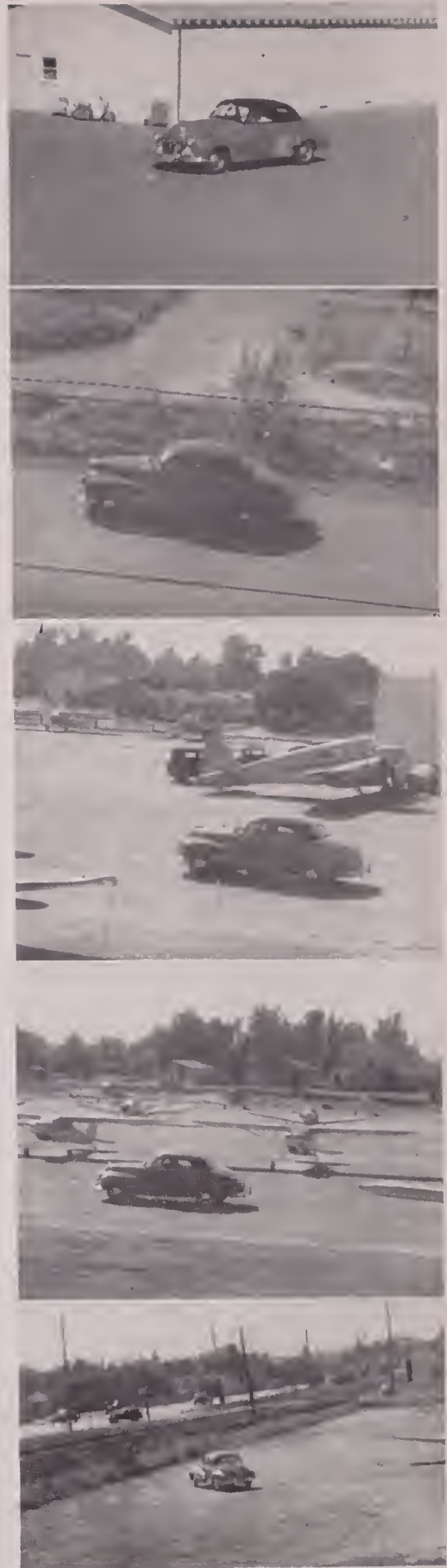
Enlarged frames from a test shot. At top, both auto and helicopter are stationary. Then the car took off across an airfield—with the camera-crane helicopter following and gradually gaining altitude. At bottom, auto has stopped, and helicopter drops down to come in for a close shot.
