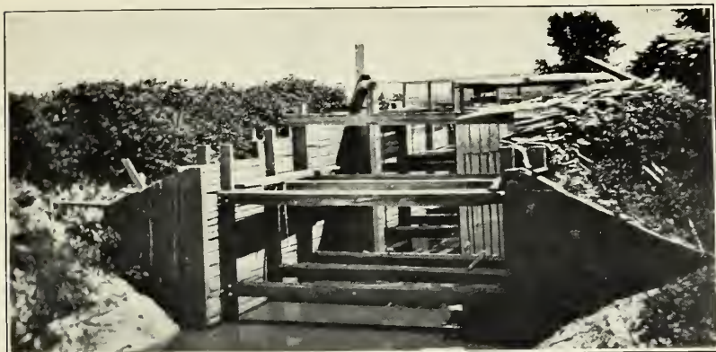
FIG. 1.—WOODEN OUTLET IN HARTWELL RANCH LEVEE.
