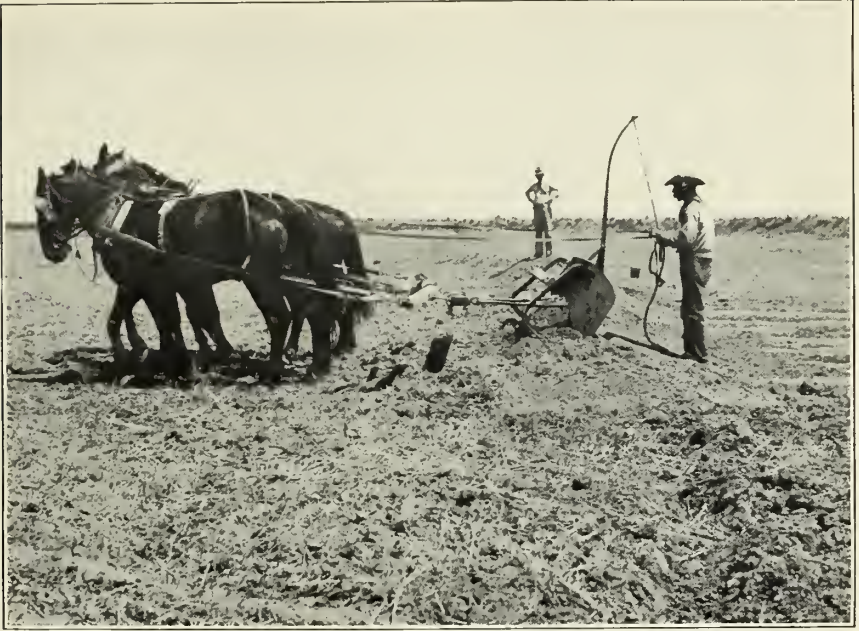
FIG. 1.—CONSTRUCTING CHECK LEVEE WITH SCRAPER.
