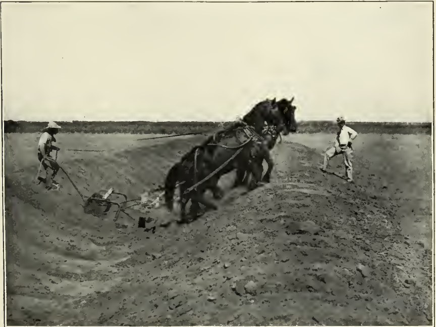
FIG. 2.—CONSTRUCTING LATERAL DITCH WITH SCRAPER.
