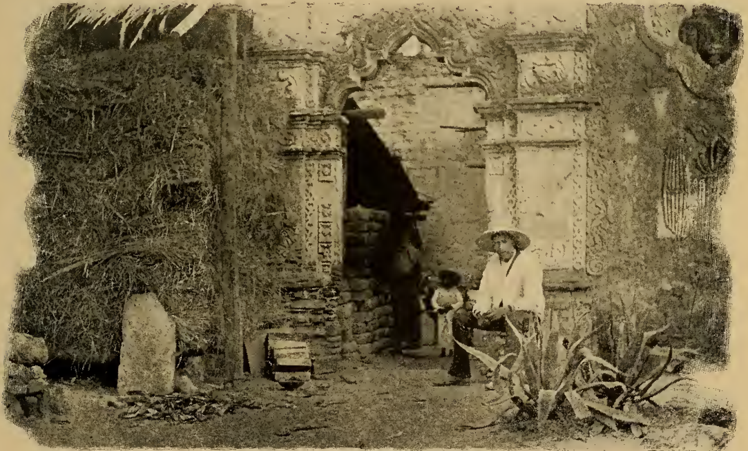
DWELLING IN A RUINED CHURCH.
