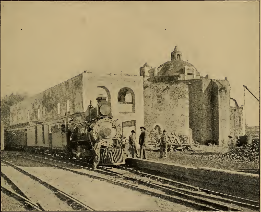
THE OLDEST RAILWAY STATION IN THE WORLD—CUAUTLA. INTEROCEANIC RAILWAY.
