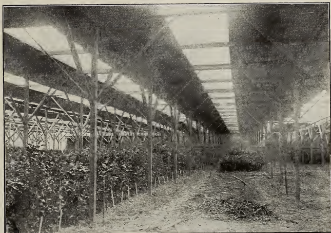
Fig. B. Interior view, showing construction. Shed erected by G. I. Taber, Glen Saint Mary Fla.
