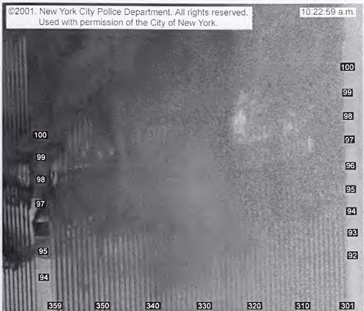
Figure 6–45. Aerial view of the south face of WTC 1 shortly before collapse.
