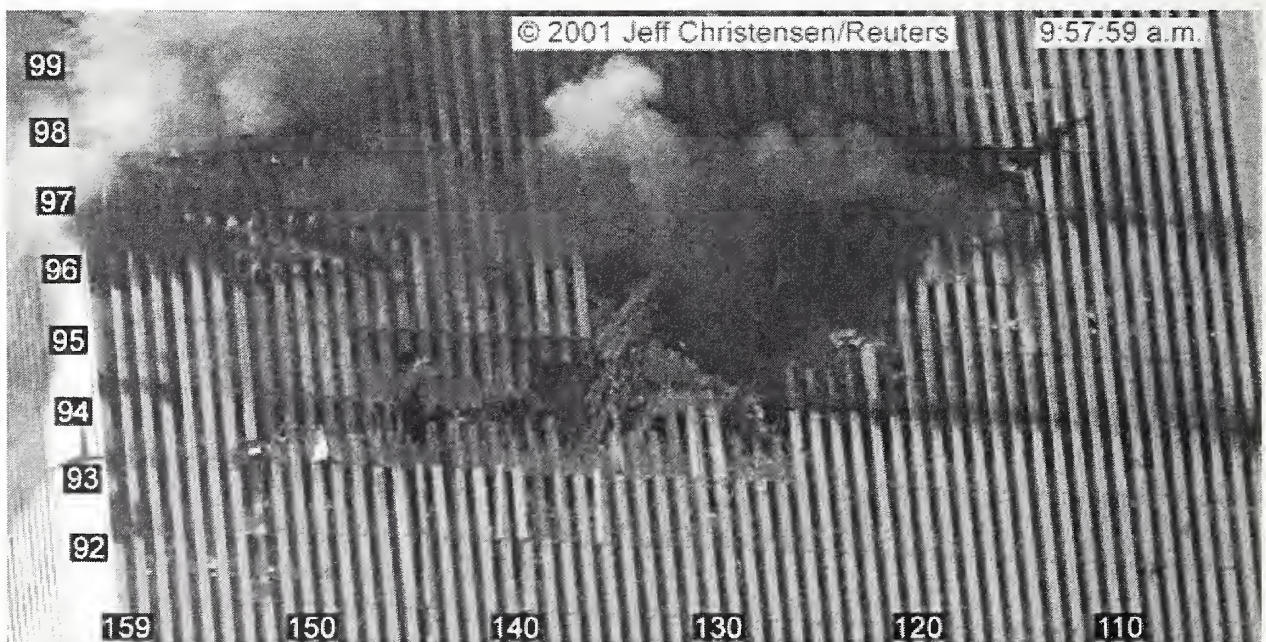
Figure 6–2. North face of WTC 1 with fires seen just inside northeast corner of floor 92.
