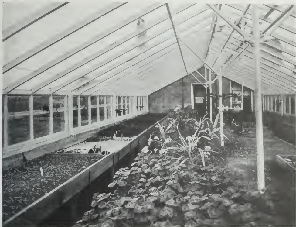
The finished house, shown in process of construction on the preceding page
