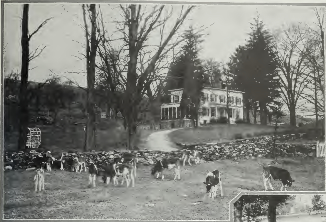
View of the master's house pleasantly situated on the hillside overlooking the dale.
