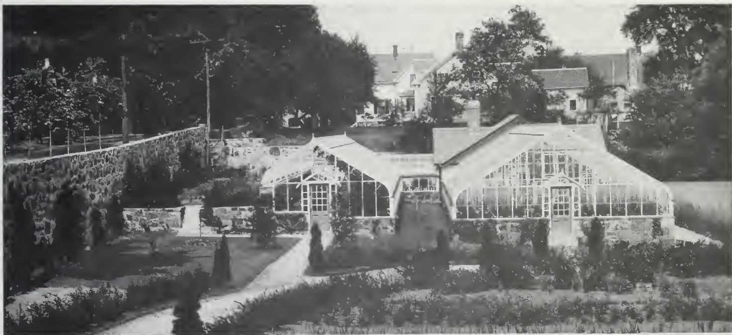
An attractive range of curved eave iron frame greenhouses for a country estate. The service building is located centrally between two even span houses (only one of which is visible), and a small connecting house joins the uneven span house to the north
