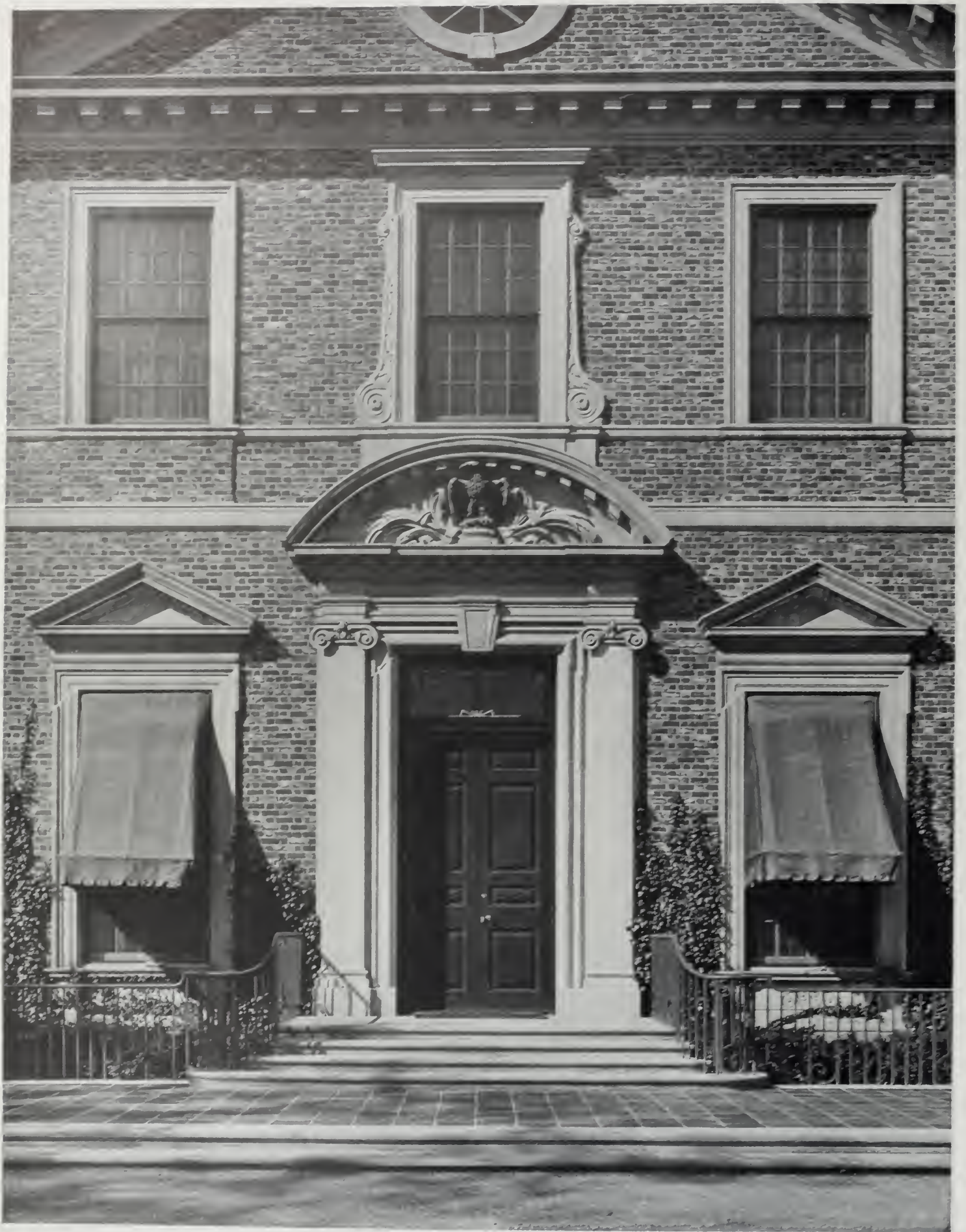
The main doorway, surmounted by an antique eagle and with its Ionic pilasters of limestone and its graceful iron railing, is an architectural masterpiece in itself. Something of the texture of the brick can be judged from this photograph
