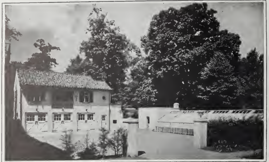
Service yard, greenhouse, stable and garage with chauffeur's and gardener's quarters
