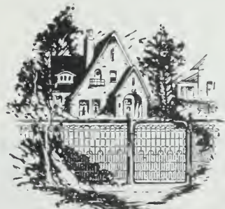
Cyclone "Complete Fence," built to measure.
