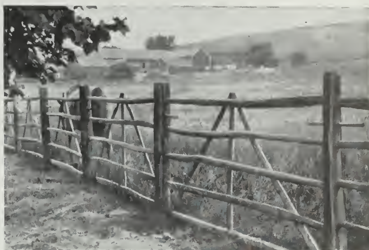
Hurdles are 8 ft. 3 in. long, with 6-ft. posts. When set, fence is 4 ft. high
