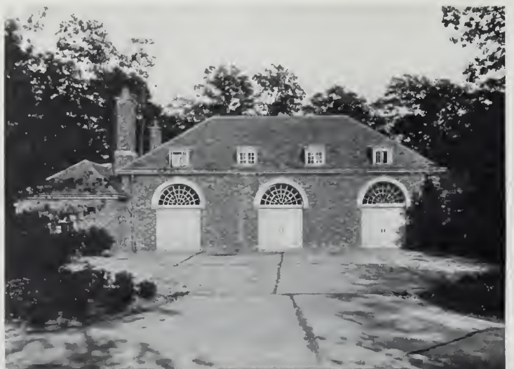
The upper level of the garage, which is built on two levels, will accommodate about twenty cars. Behind the garage is a detached house with quarters for visiting chauffeurs
