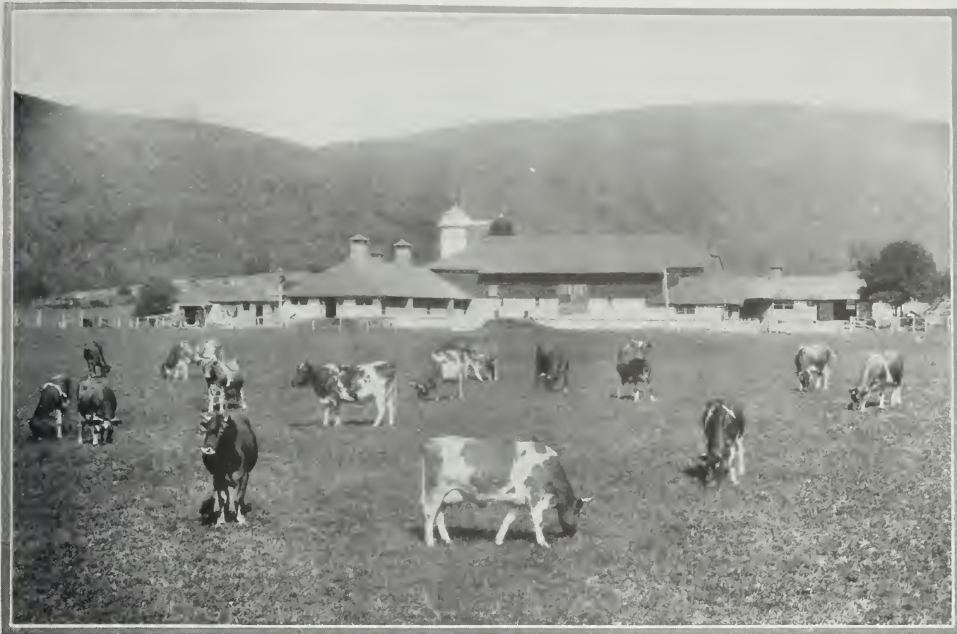
Group of dairy buildings designed by Alfred Hopkins and built of concrete, hollow tile, and shingles. It accommodates a breeder's herd of thirty-eight cows with bulls, young stock, etc., a total of seventy head.
