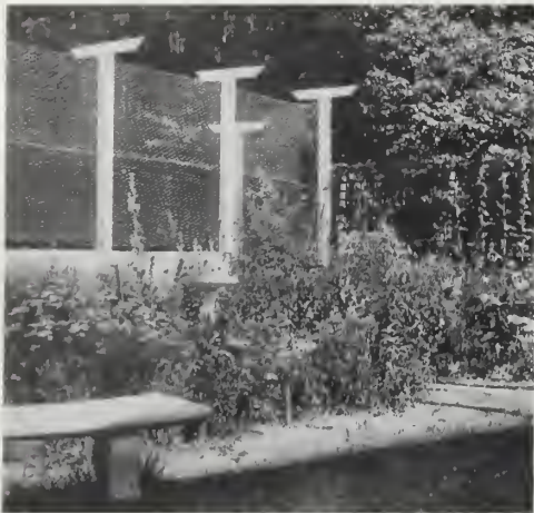
Showing a section of the cement wall which serves simultaneously as a background for the garden and retaining wall for the tennis court
