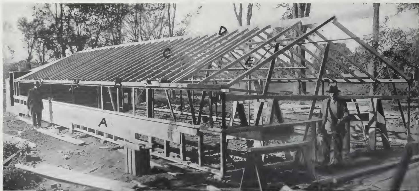
The same house pictured above, as it looks from the outside. A is the wooden side wall resting on the concrete foundation piers. B is the eave
