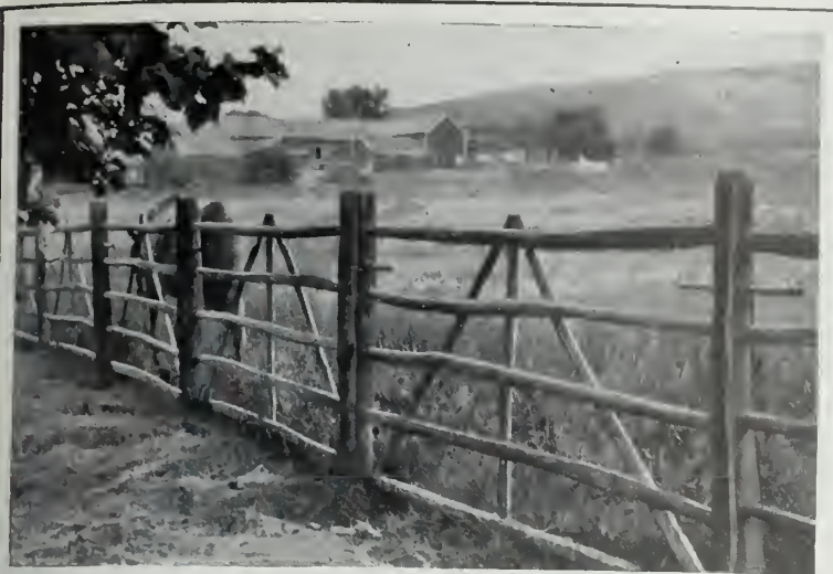
Hurdles are 8 ft. 3 in. long, with 6-ft. posts. When set, fence is 4 ft. high
