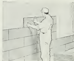
Armstrong's Corkboard is easily erected in any type of construction—brick, stone, tile or frame. It is furnished in boards 12 by 32 or 36 inches from 1 to 3 inches thick.
