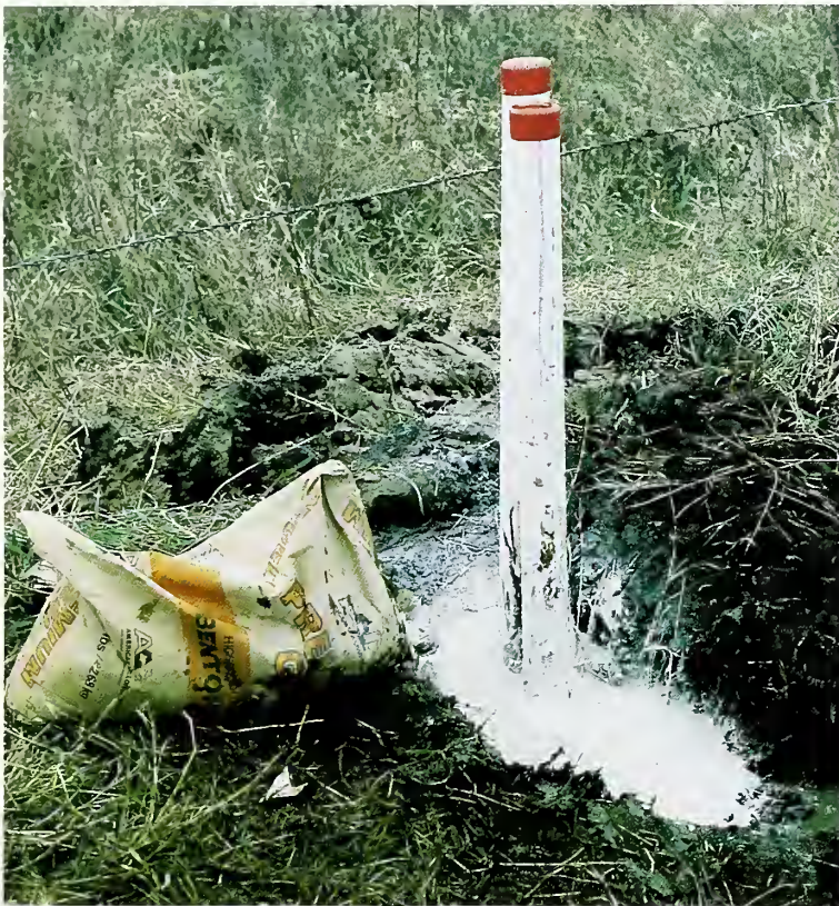
Figure 8. Bentonite seal at the land surface.
