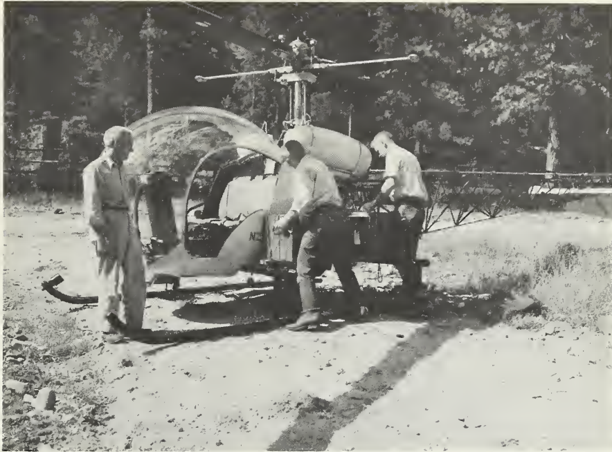
Attaching cargo to cargo racks for resupply to lookouts
