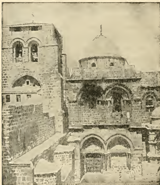
Church of the Holy Sepulchre, sometimes claimed to be built upon the site of Calvary
