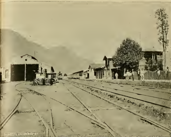
STATION OF ORIZABA. ENGINE RUNNING SHED ON LEFT.
