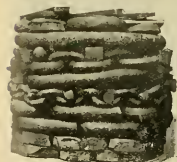
PILE OF SCRAP, READY FOR FURNACE.
