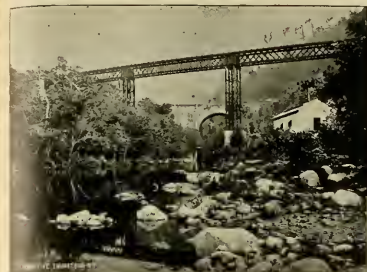
BRIDGE OF THE AHOVAL. NATIONAL HIGHWAY BRIDGE BEYOND.
