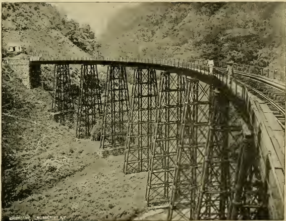
CANTON BRIDGE, BARRANCA DE METU, CURVE OF 325 FEET RADIUS, MEXICAN RAILWAY
