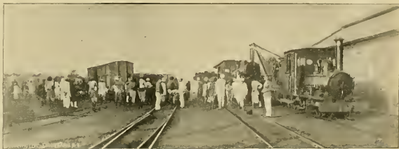
WORK ON A STATE ROAD IN INDIA.
