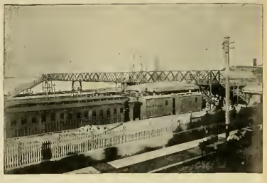
FOOT BRIDGE AT NEW CASTLE, NEW SOUTH WALES, BUILT OF OLD RAILS.
