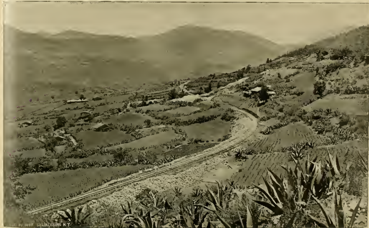
TYPICAL SCENE ON INTEROCEANIC RAILWAY, BETWEEN PUERTO AND CITY OF MEXICO. INDIAN CULTIVATION OF AGAVE, OR CENTURY PLANT.
