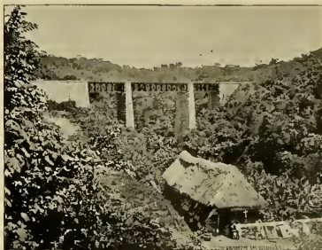
CHICAGO BRIDGE, MAIN IN RAILWAY.
