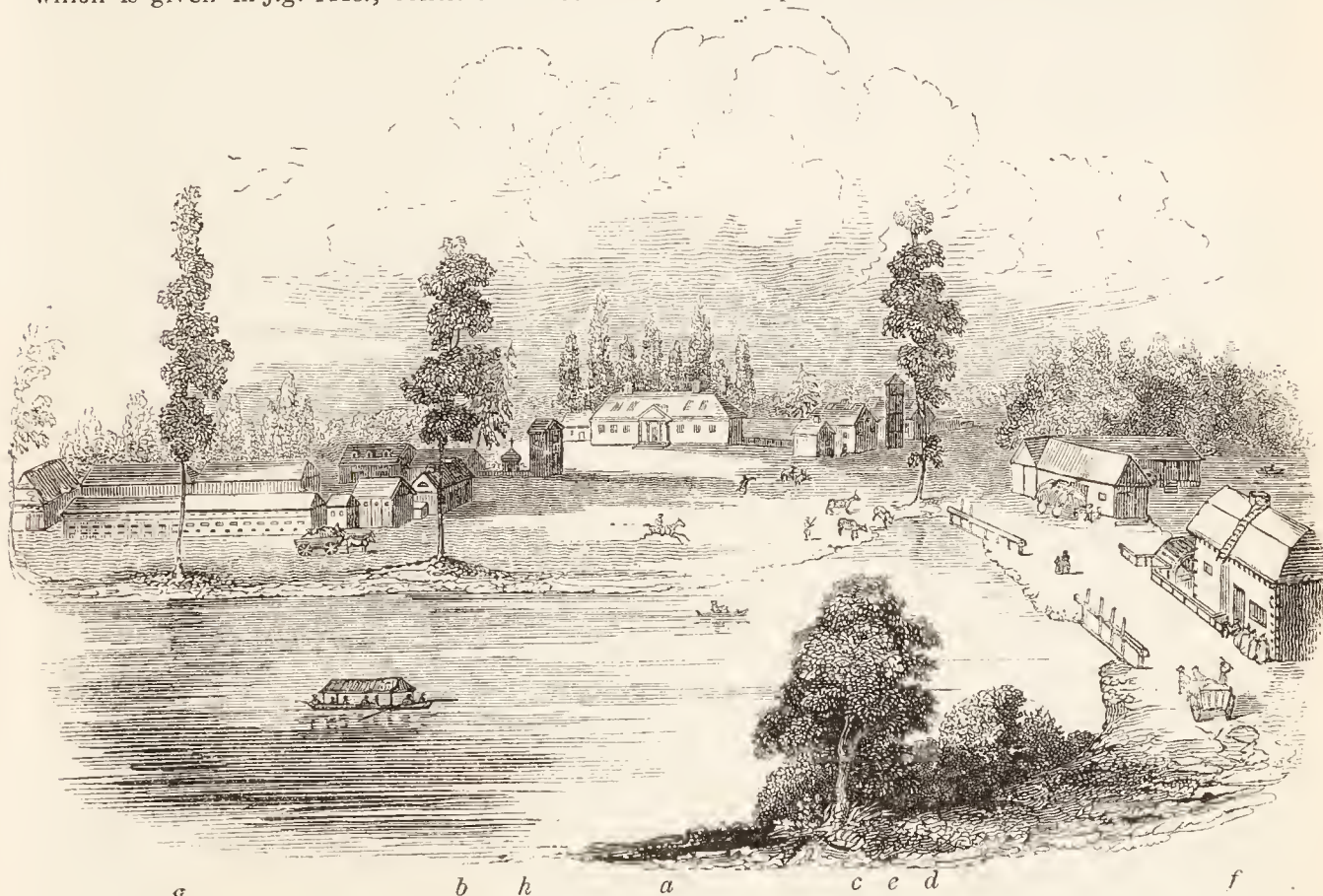
in 1832. The buildings consist of a dwelling-house ( a ), with a detached kitchen ( b ), a brewery ( c ), a distillery ( d ), a machine for raising water to supply both ( e ), a corn-mill ( f ), sheds for feeding cattle ( g ), an ice-house ( h ), in which ice is kept above ground by means of thick double walls and doors; and large barns, a threshing-machine, coach-house, stabling and all other offices, including a carpenter's shop and house, blacksmith's shop and house, bailiff's house, &c. Besides these there is a small colony of cottages for the common labourers. These cottages are generally of the kind called log houses, and, with their draw-wells attached, present the appearance of fig. 1149. The Germans who are settled in Poland, as agricul-
