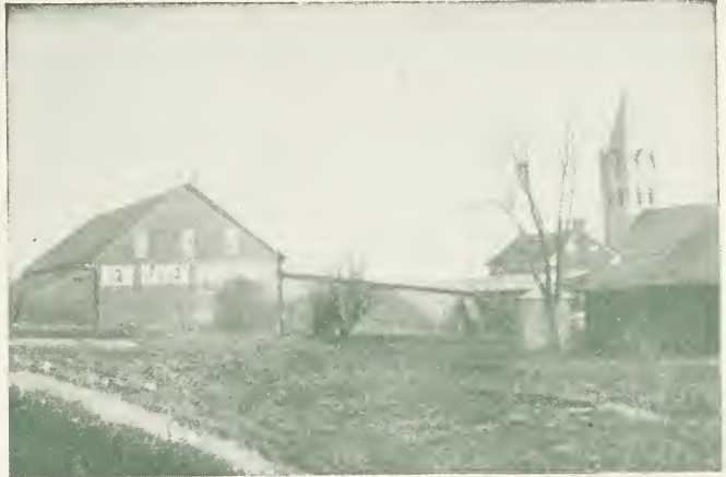
View of Our Storage Sheds
