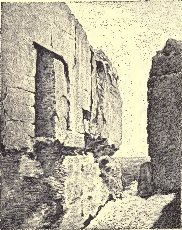
FIG. 4. EAST WALL OF NORTH ROOM
