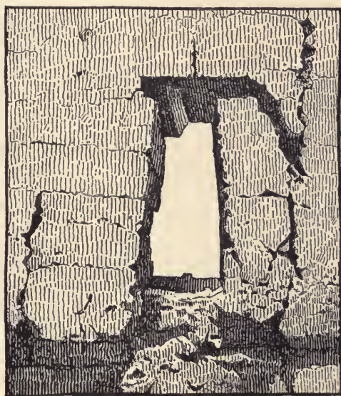
[Fig. 5. NORTH WALL OF NORTH ROOM
