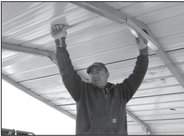
Loyd Bantz steadies the new shelter at Payola reservoir.
