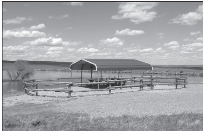
The newly constructed picnic shelter at Payola Reservoir.
