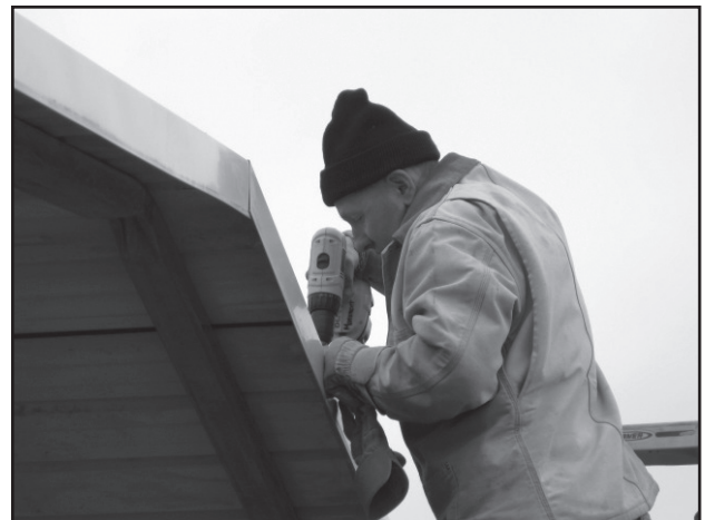
Mike Barrick installs an end cap on the shelter.
