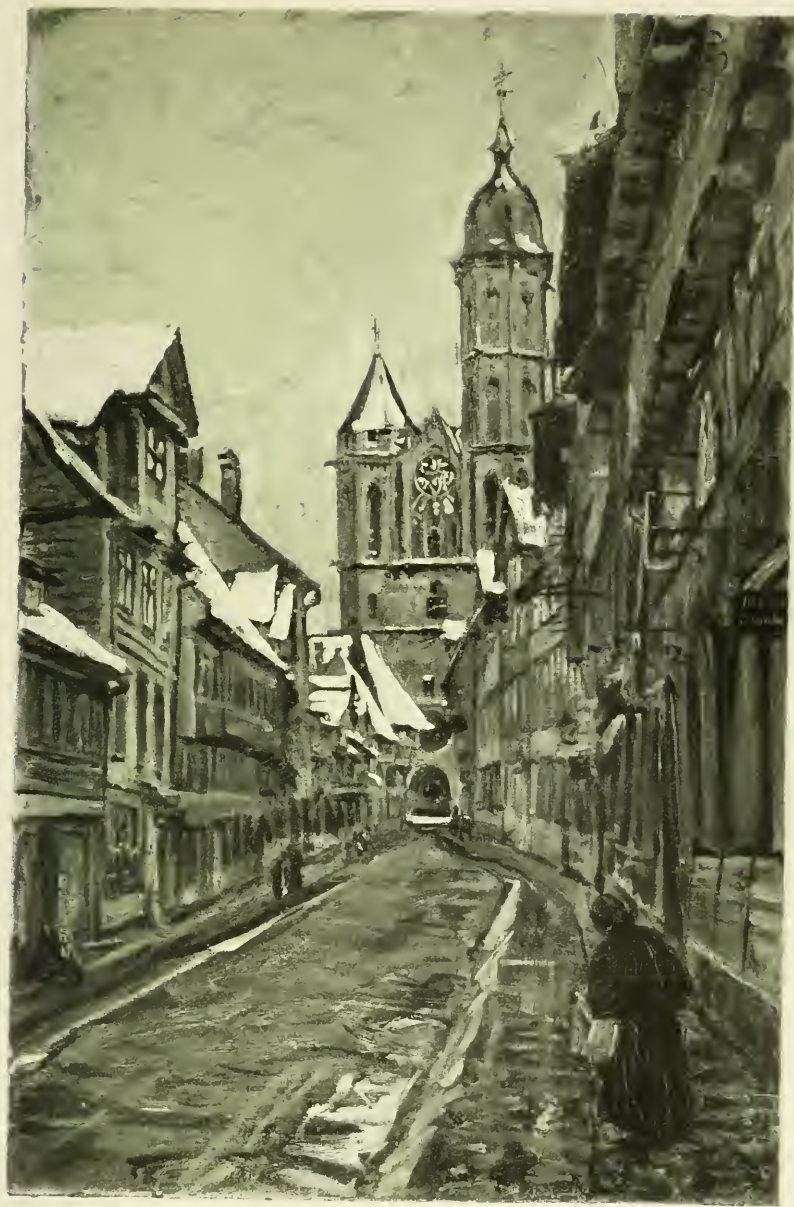
THE FRONT OF ST. ANDREW'S, AS SEEN FROM THE WEBER-STRASSE
