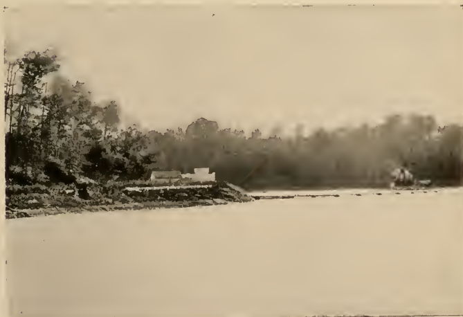
Baltimore's Water Supply — Loch Raven Reservoir
