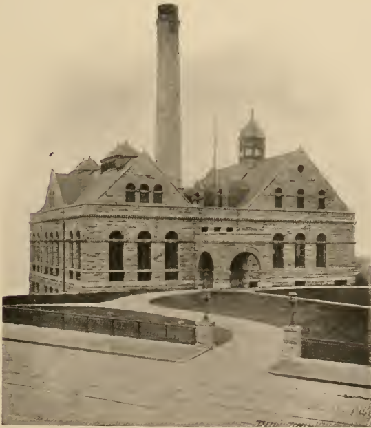
Baltimore's Water Supply — Mt. Royal Pumping Station
