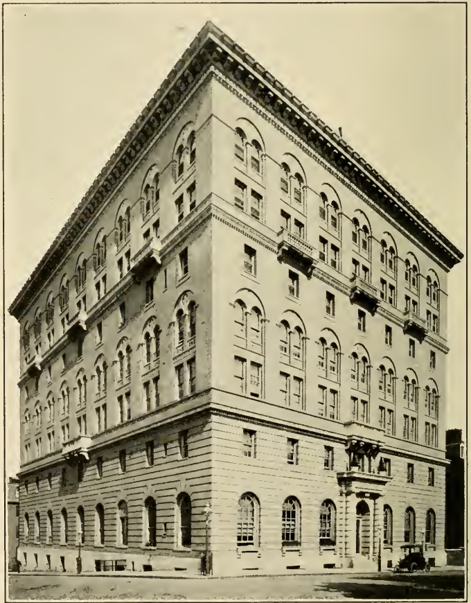
Y. M. C. A. BUILDING—FRANKLIN AND CATHEDRAL STREETS
