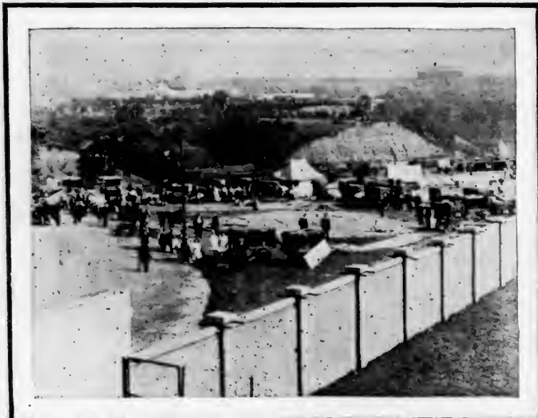
After the blow-down at Pittsburg, Pa., Labor Day.
