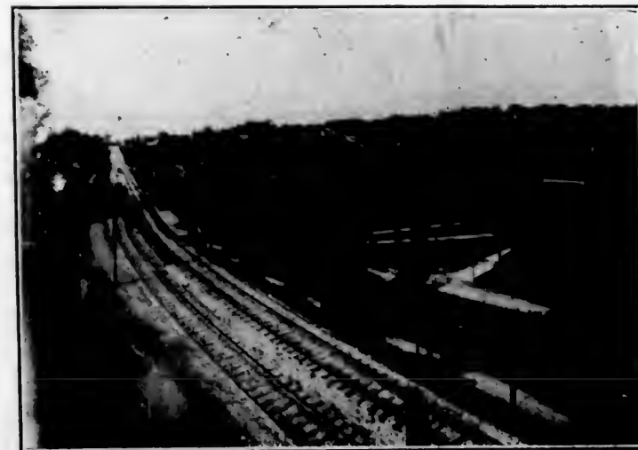
View of Car Line Exit from Grounds.
