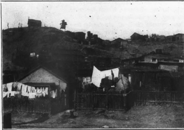
HOUSE BUILT TO SUIT THE WISHES OF ITALIAN LABORERS
