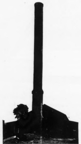
Chimney built for the E. G. Hill Co., Richmond, Ind.
