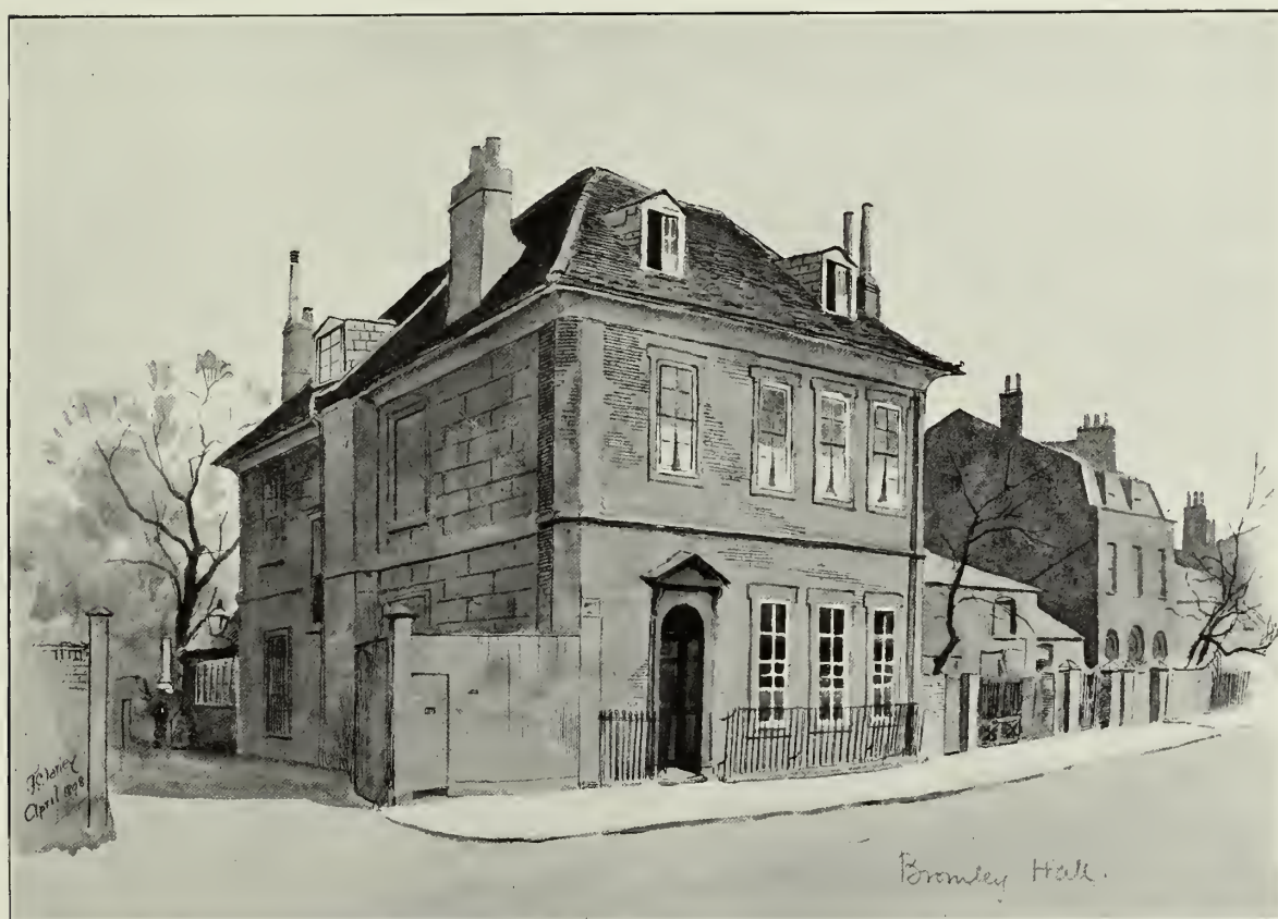
VIEW FROM NORTH-WEST, WITH THE "MANOR HOUSE" ADJOINING.
