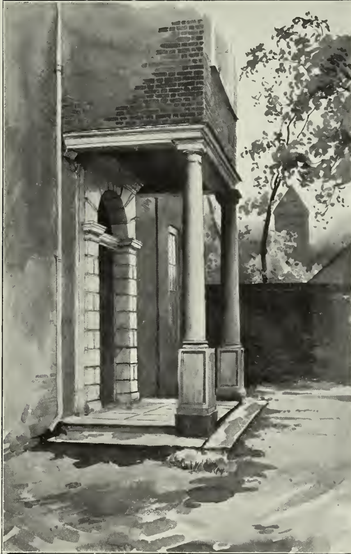
PORCH FROM SOUTH SIDE.
