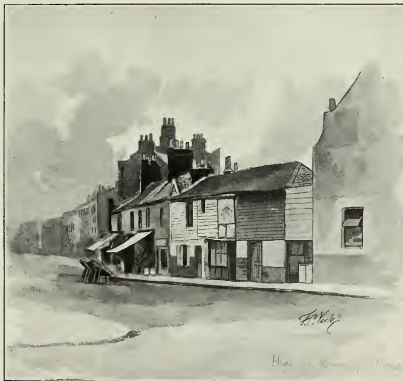
VIEW FROM NORTH-EAST
