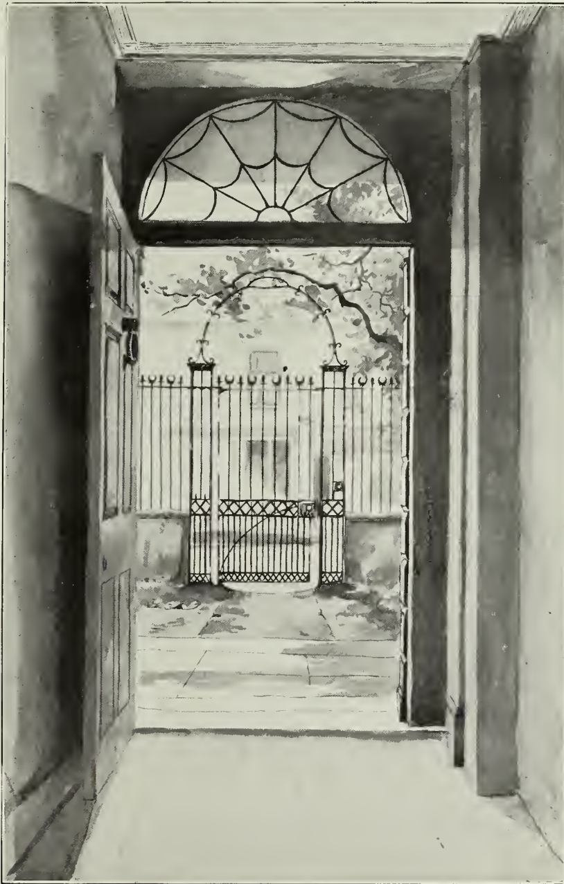
ENTRANCE DOOR AND RAILINGS IN FRONT.
