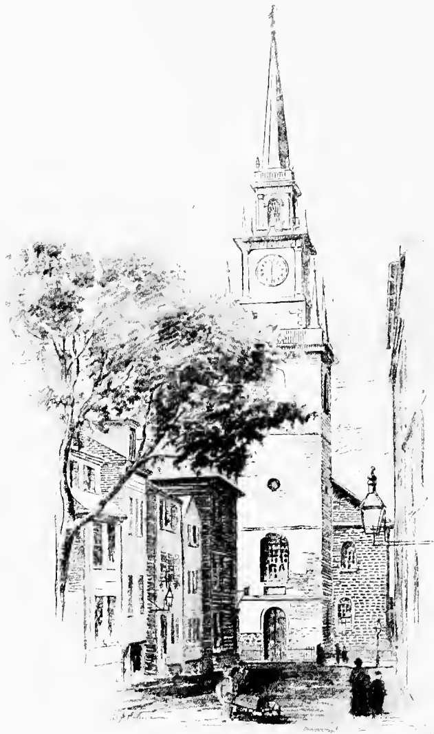
THE OLD NORTH CHURCH (From which Paul Revere's signals were displayed.)
