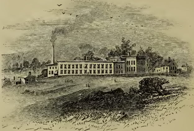
APPEARANCE OF THE OLD FACTORY.
