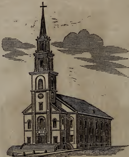
HOLLIS-STREET CHURCH—Hollis street.
