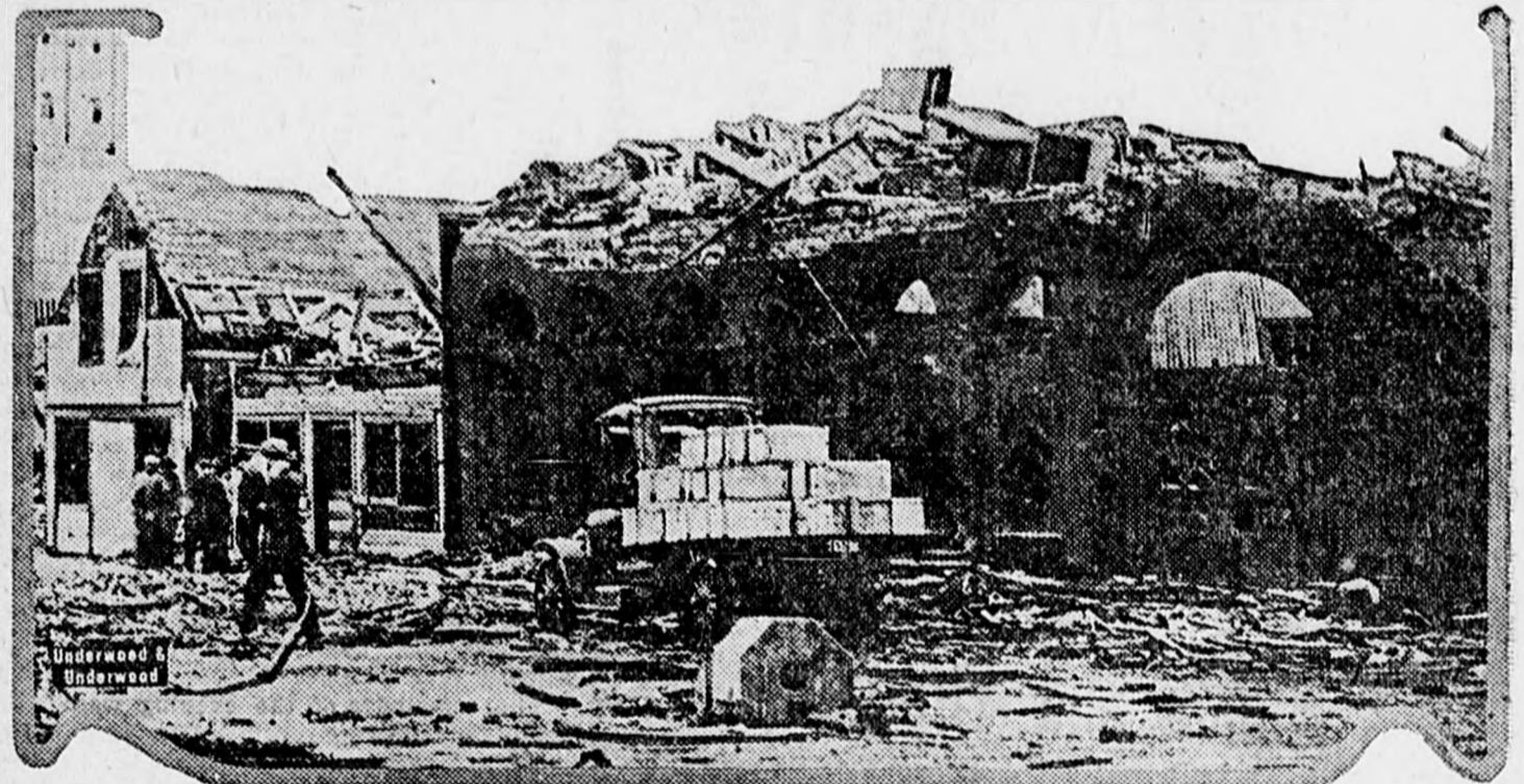
Ruins of business buildings on Union avenue, Fergus Falls, Minn., destroyed by a tornado that killed several hundred persons and wrecked much of the town.
