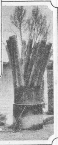
B. Simple apparatus for end treatment.
