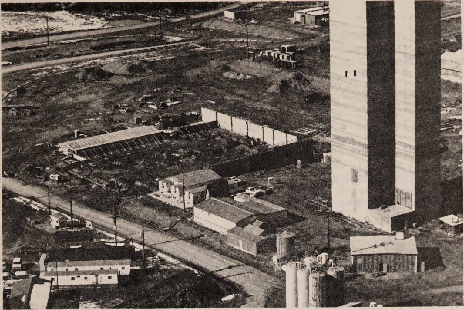
Figure 4-30. Aerial view of construction near the headframes. (October 1981)
