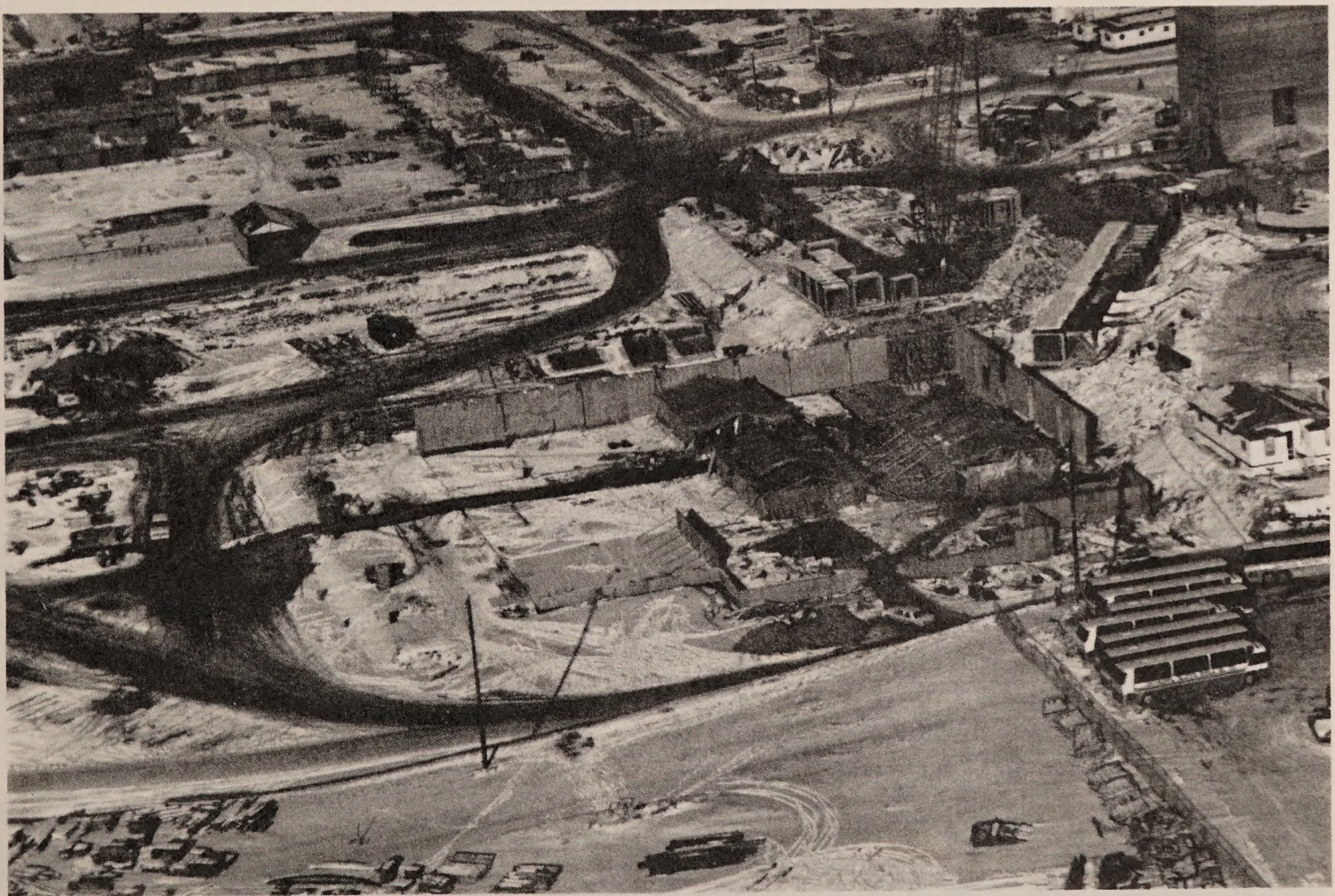
Figure 4-21. Aerial view of changehouse and tunnel construction. (November 1981)
