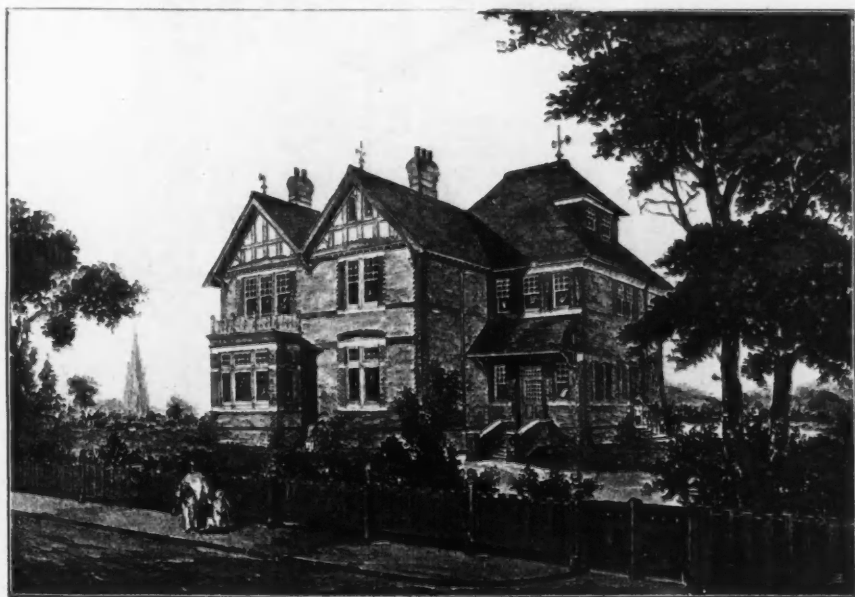
Villa Residence, Surbiton Hill, for R. A. Morris, Esq., J.P., J. BUCKLEY WILSON, F.R.I.B.A., AND T. E. LIDIARD JAMES, M.S.A., Architects. (For plans see p. 146.)
