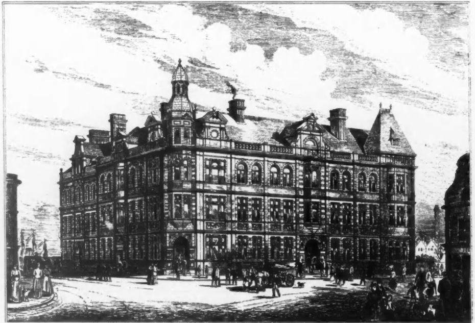
New Bank and Suites of Offices, Goole, for Messrs. Beckett and Company, HENRY B. THORP Architect.
