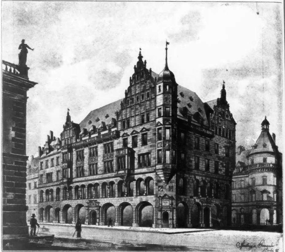
Business Premises in Dresden, SPALDING AND GRENANDER, Architects, Berlin.
