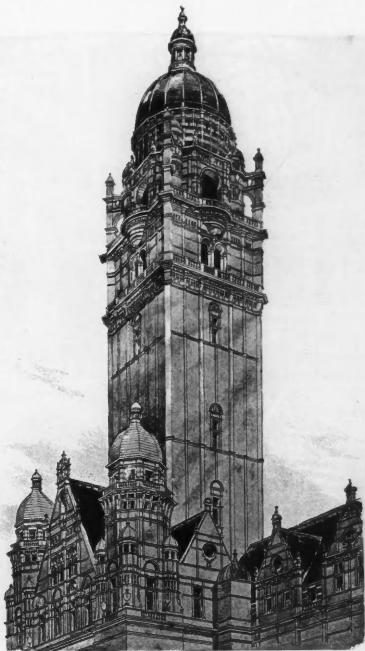
1644. The Queen's Tower, Imperial Institute , THOMAS E. COLLCUTT, F.R.I.B.A., Architect.
