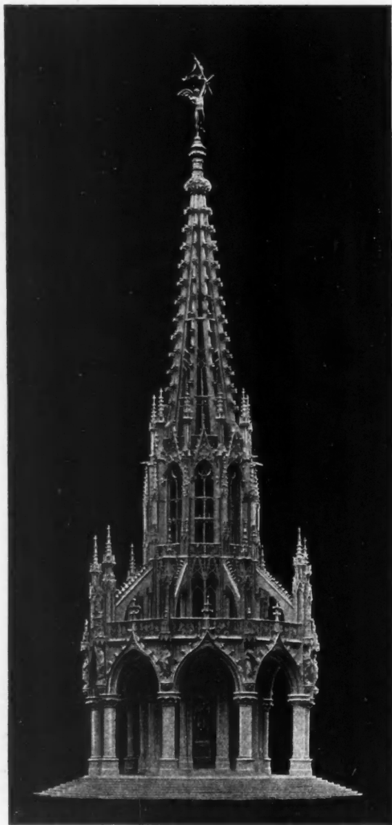
Memorial to His late Majesty Leopold I., King of the Belgians, erected in front of the Palace at Laken, near Brussels, LOUIS DE CURTE, Architect, Brussels.
