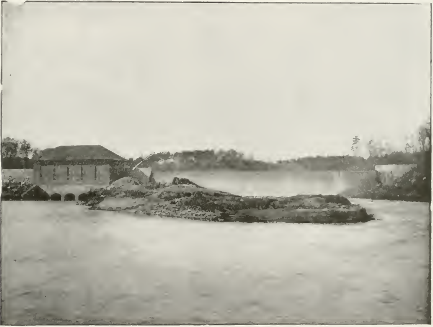
Water Power on Saluda River at Pelzer, South Carolina
