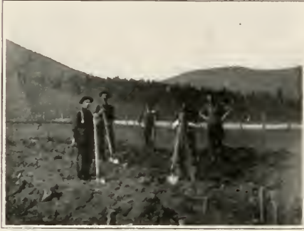
Brecking Ground for Nursery at Asaph, Pa.
