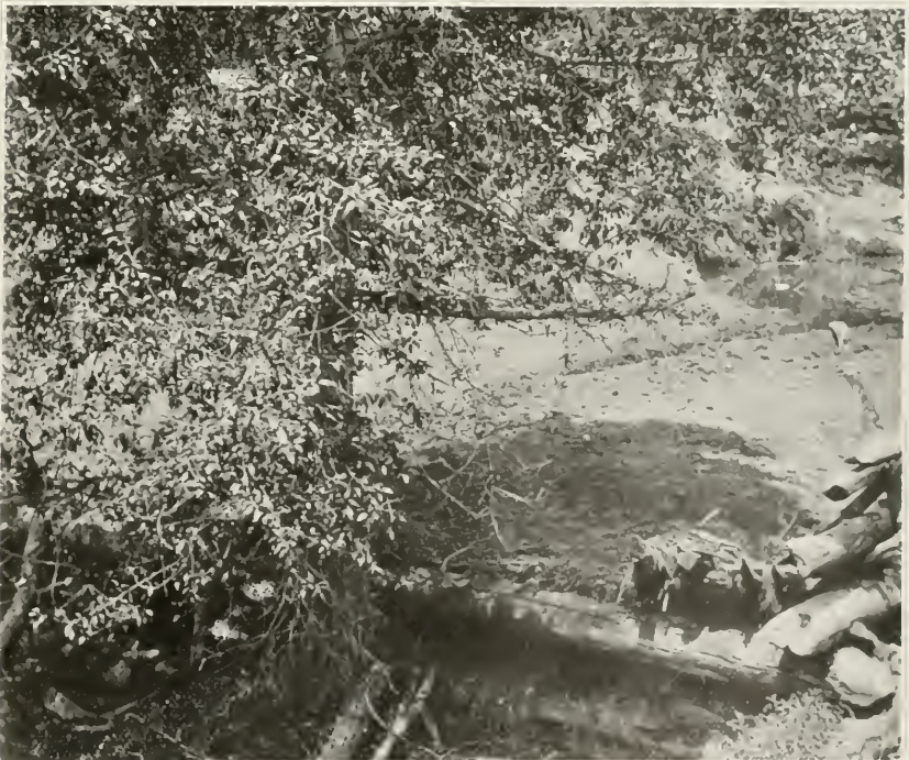
Dam filled with silt, in the Tonto Basin, Arizona—Tonto National Forest will prevent such occurrences in future
