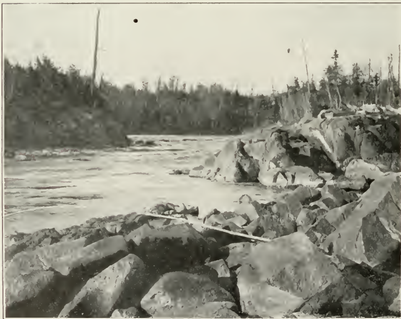
View of Dam Site on Flambeau, Tributary of Chippewa River, Wisconsin, at Big Falls
