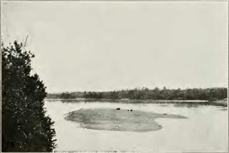
DESTRUCTION OF A WATERWAY Formation of Silt Bar in a Navigable Stream
