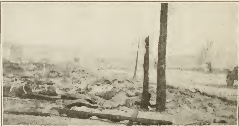
ANOTHER VIEW IN CHISHOLM, AFTER THE FIRE
