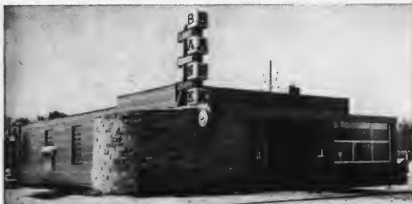
ULTRA-MODERN SUBURBAN Lake County State Bank uses a 100% National System.
