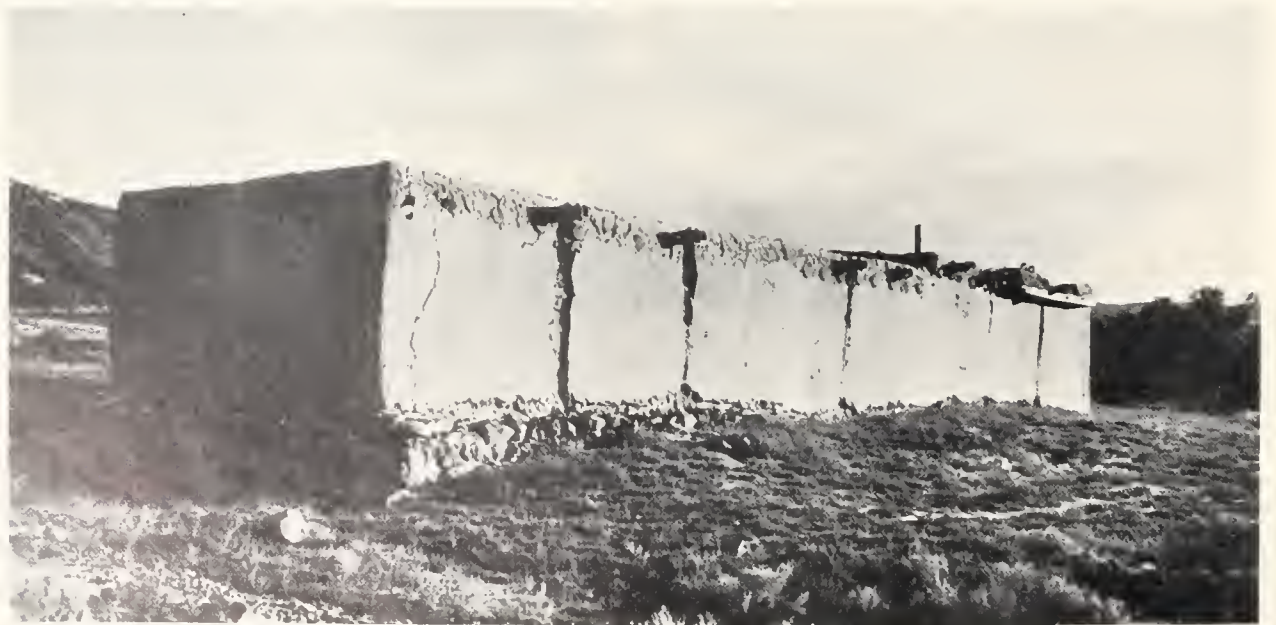
FIGURE 6. EAST Morada . SIZE: 28.82 meters long, 4.88 wide, 3.58 high. DATE: 19th century. LOCATION: 300 meters east-southeast of Santo Tomás Church in main plaza; seen from northeast corner. MANUFACTURE: Adobe bricks set on stone foundation; wood drains ( canales ) and beam ( viga ) ends at top of wall.
