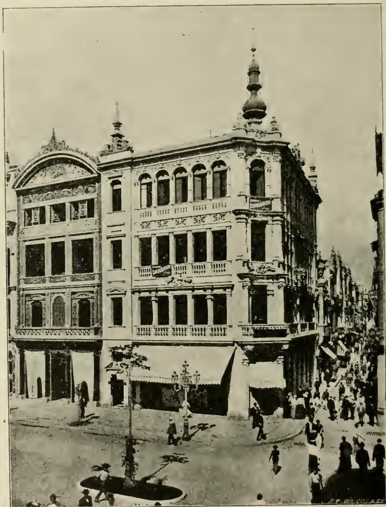
Rio. — New Buildings
