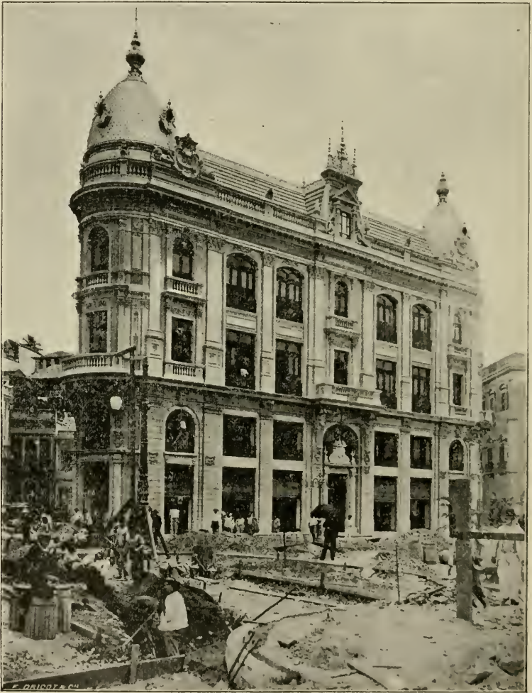
Rio. — New Buildings
