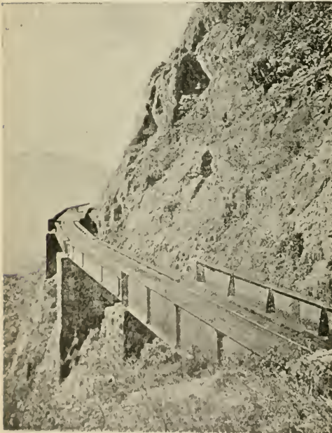
ENGINEERING WORKS IN BRAZIL. — The celebrated Carvalho Viaduct on the Parana Railway.
