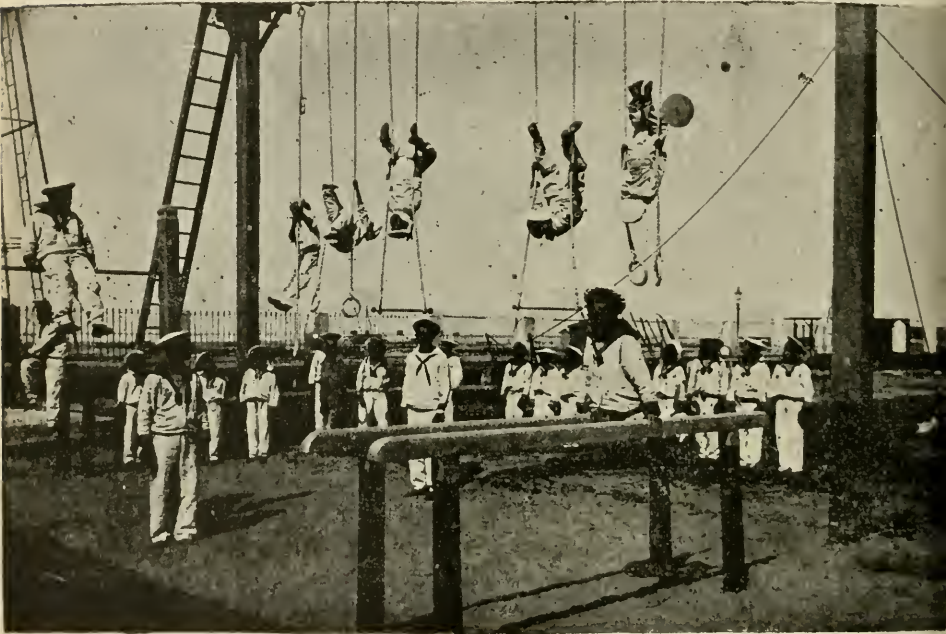
Fortaleza. — Gymnastic-room of the Marine Apprentices School
