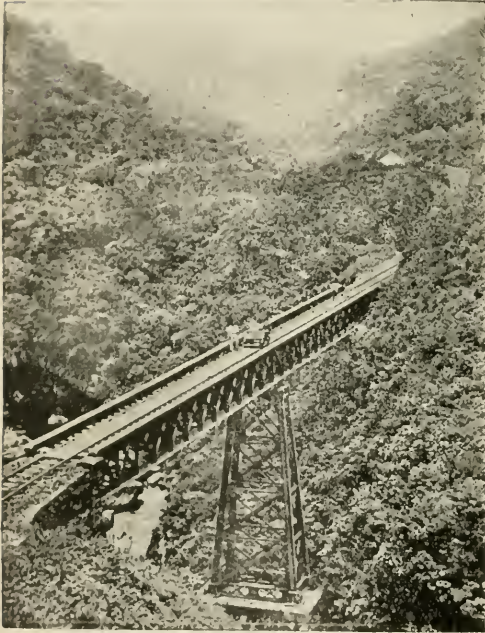
ENGINEERING WORKS IN BRAZIL. Bridge over the rio Ypiranga, in Parana.
