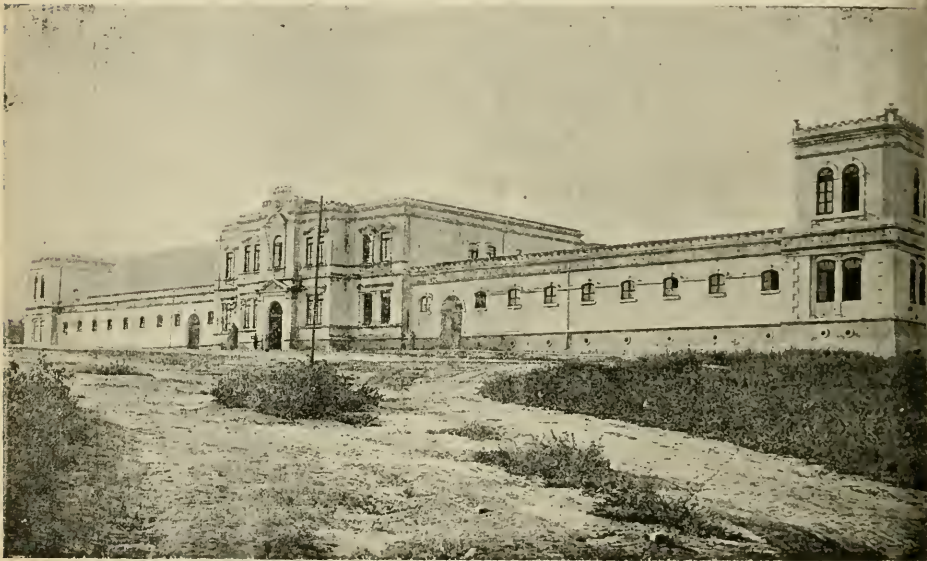
Belo Horizonte. — Barracks of the Public Force
