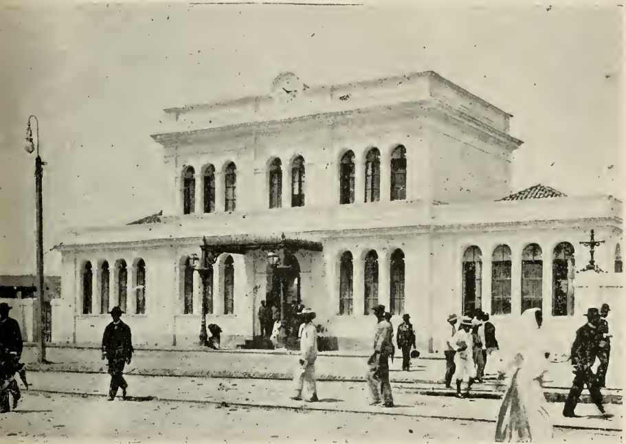
Maceió. — Principal railway station
