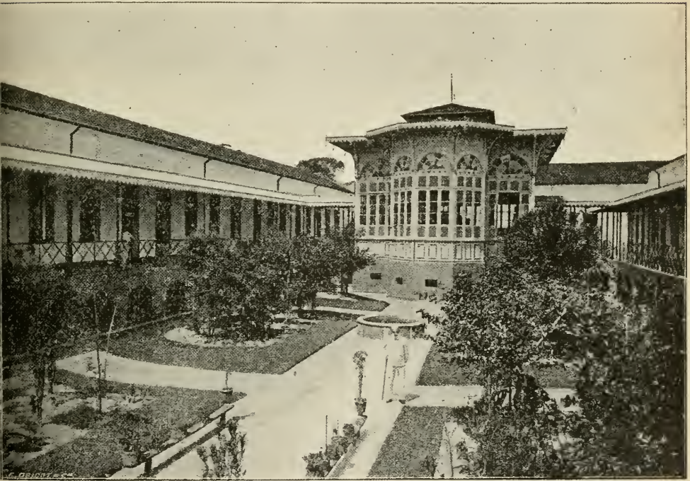
Belem. — Asylum for the poor. Interior Garden and Refectory; Men's Side
