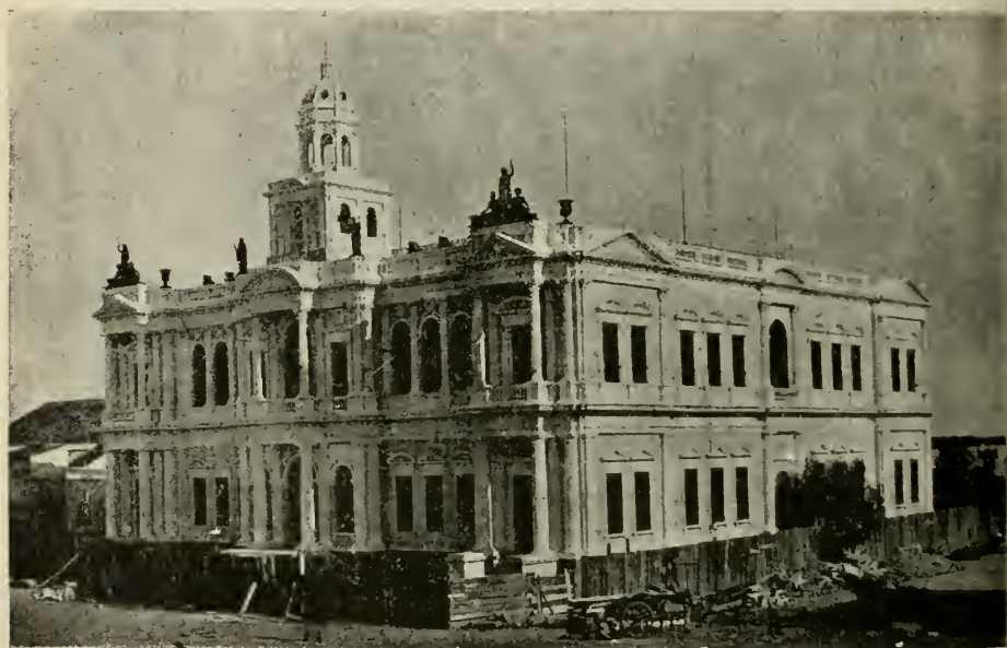
Porto Alegre. — Municipal building
