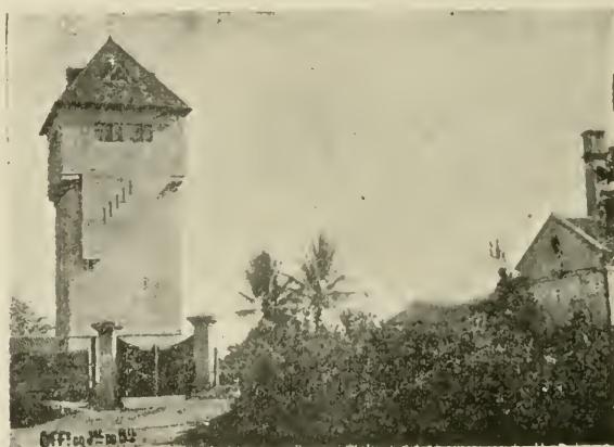
Campos. — Water reservoir
