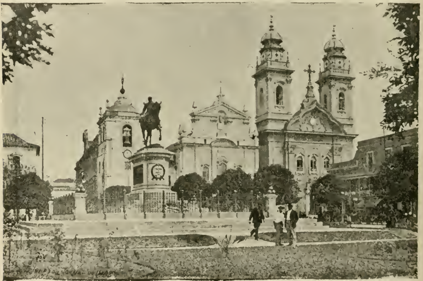
Rio. — The Cathedral and do Carmo Church
