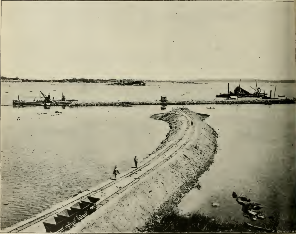
Port of Rio. — Filling up of the Sea Zone
