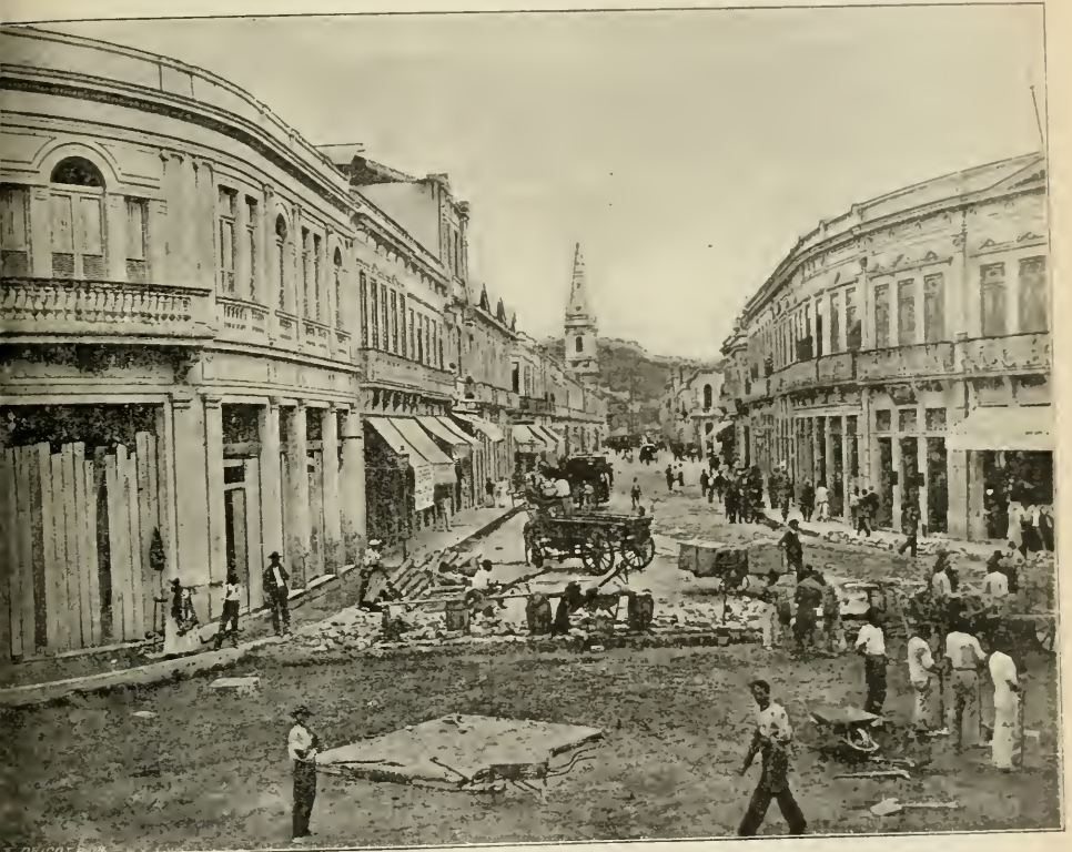
Capital Federal — Construction of the Passos street
