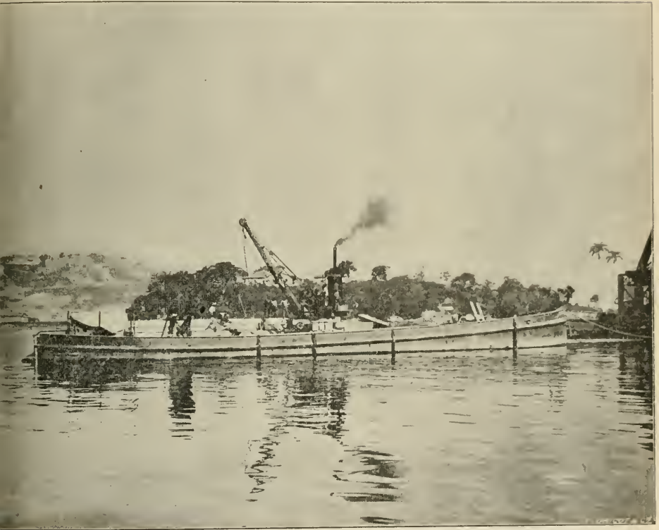
Port of Rio. — Construction of the New Quay. Crane-boat
