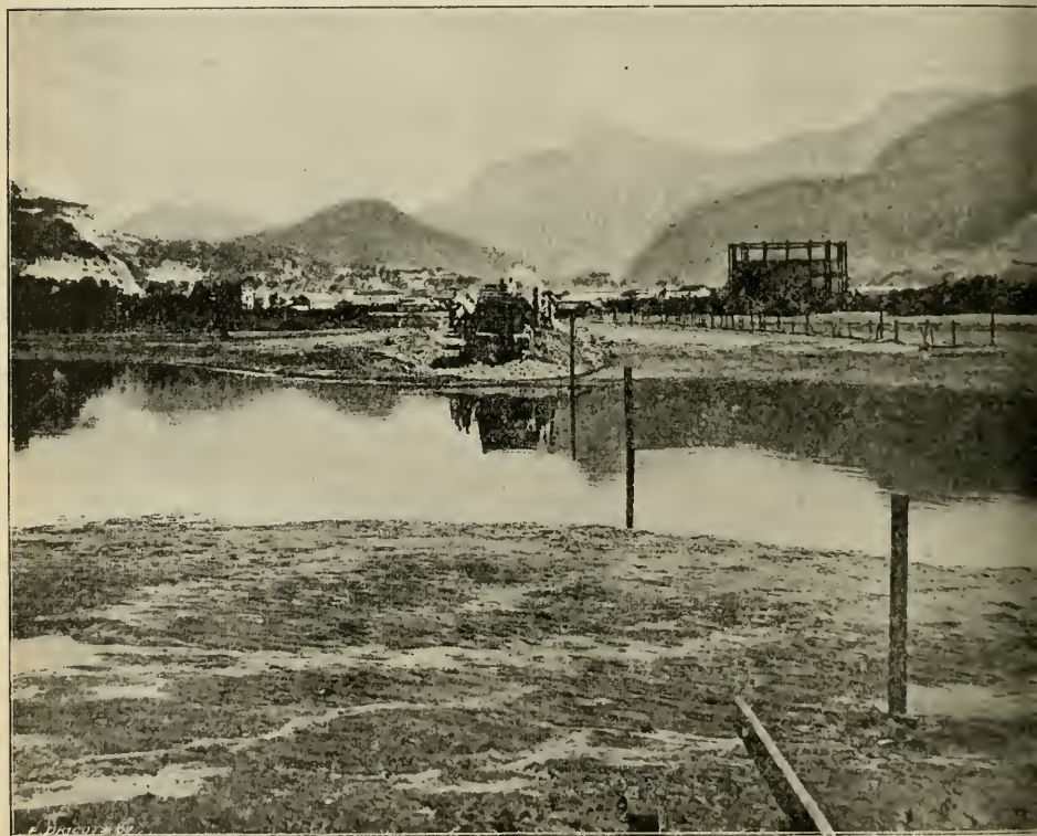
Port of Rio. — Filling up of the Sea Zone
